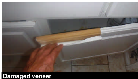
Damaged veneer
