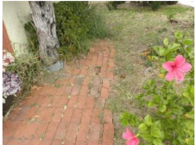
Uplifted and dislodged bricks in the south yard at unit 1.
