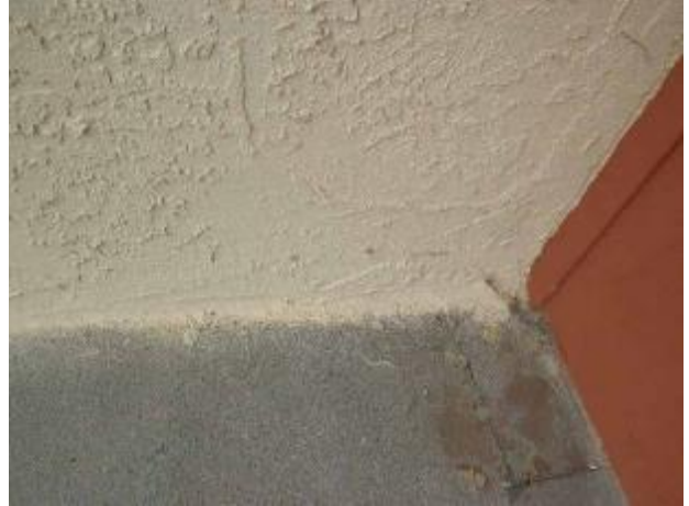
Example of wrong material for water proof decks, no flashing installed, and splits/cracks in the material.
