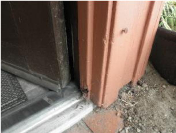
Moisture damage to the base of the jamb at the front entry door in unit 1.
