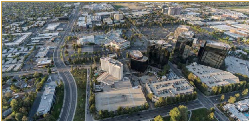
Warner Center — ¼ Mile East of Subject
