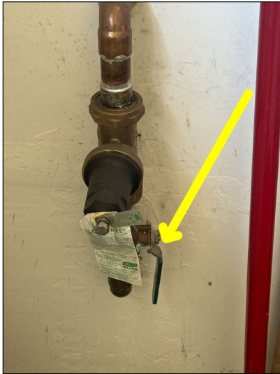
Main water shut off to the home where the main water line enters the home.
