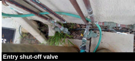
Entry shut-off valve
