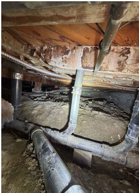
Substructure: Sub floor material Wood Planks Subfloor
