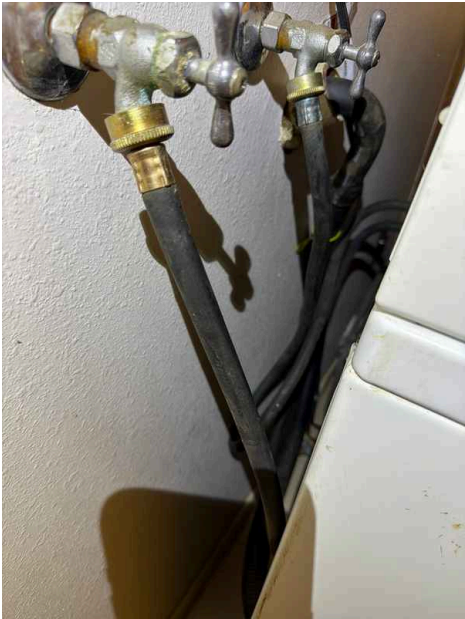
Clothes Washer: Supply Hose Type Rubber
