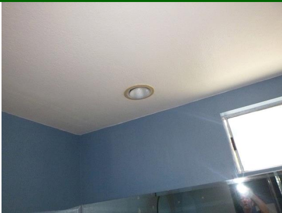
2nd Floor Bathroom:
