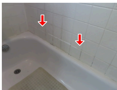
6.7 Item 2(Picture) hall bathroom
