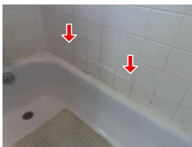
6.7 Item 2(Picture) hall bathroom
