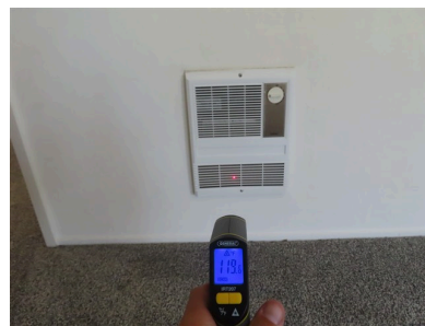
5.0 Item 2(Picture) bedroom 1
