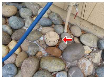
1.1 Item 1(Picture) lower front of building
