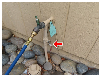
1.0 Item 1(Picture) lower front of building
