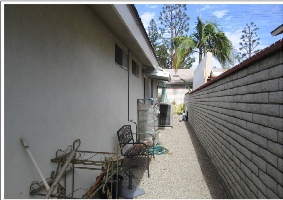
Side View of Subject Property (east)
