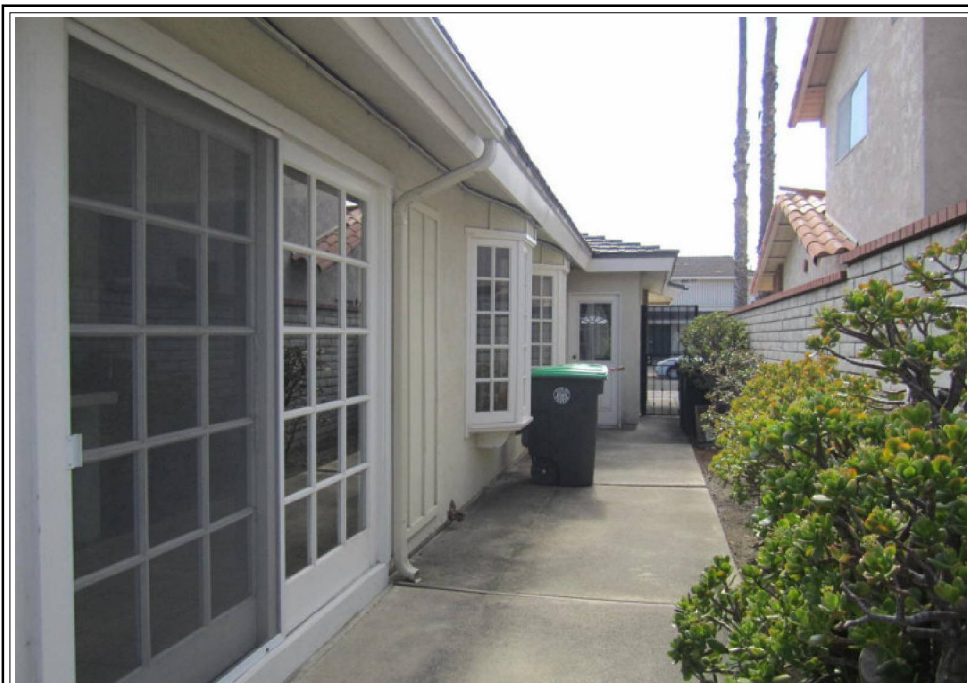
Side View of Subject Property (west)
