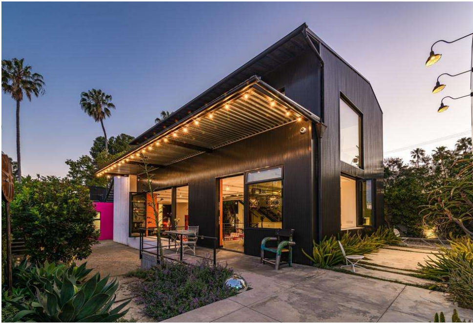
The home's distinctive shell was modeled after a combination of Santa Monica's Bergamot Station Arts ... [+] HILTON & HYLAND
