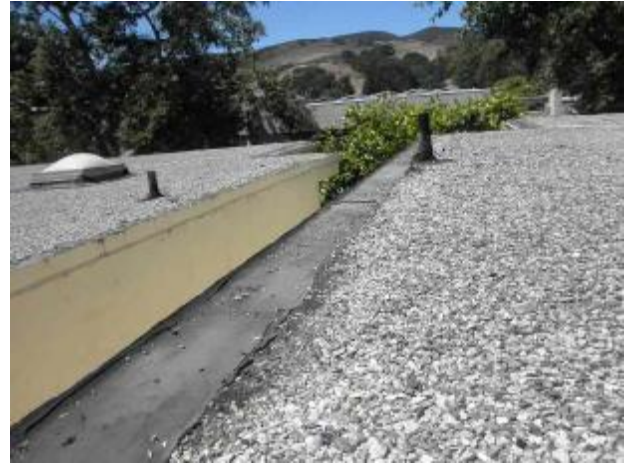
Patching along the perimeter of the tar & gravel roofing.
