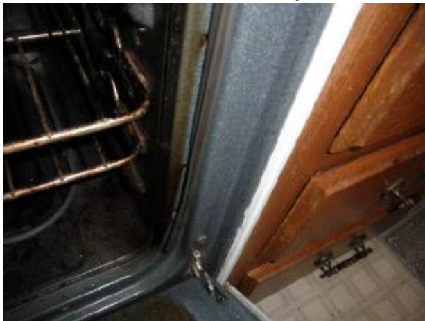
Damaged door gasket at the oven in unit 3.
