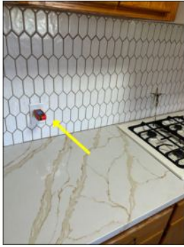
Outlet hot wired in reverse with neutral - needs to be serviced
