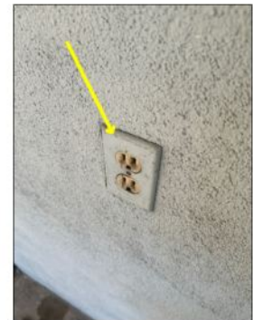
Exterior outlet/switch covers are missing or not of proper exterior weather proof type - needs to be serviced
