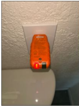
Outlet hot wired in reverse with neutral - needs to be serviced - garage
