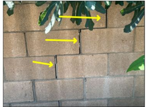
Cracking large/separation cracks present - needs to be serviced
