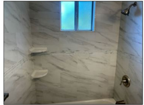
Shower walls have normal wear for age at the time of the inspection - no major visible defects - recommend routine grout and sealer maintenance
