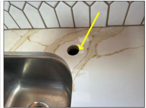
Missing cap - needs to be serviced
