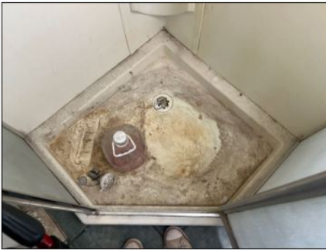
Shower pan is in a worn/stained/older condition - typical for the age - recommend routine grout and sealer maintenance
