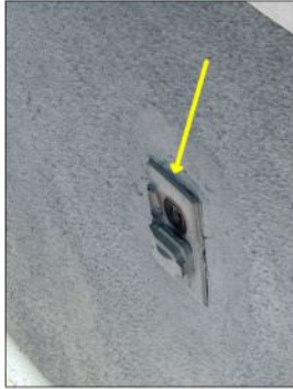
Exterior outlet/switch covers are missing or not of proper exterior weather proof type - needs to be serviced
