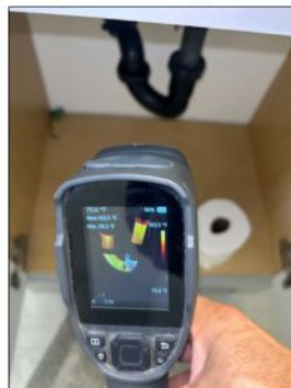
Thermal Image View
