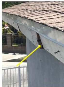
Warped wood / twisted wood - signs of age and wear - recommend servicing
