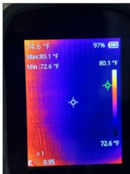
Temperature at Air Return
