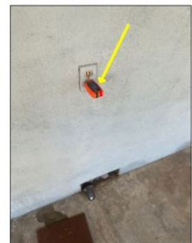
Outlet hot wired in reverse with neutral - needs to be serviced
