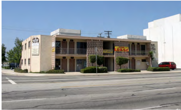
Office Space For Lease 800/SF @ $2.09/SF MG
