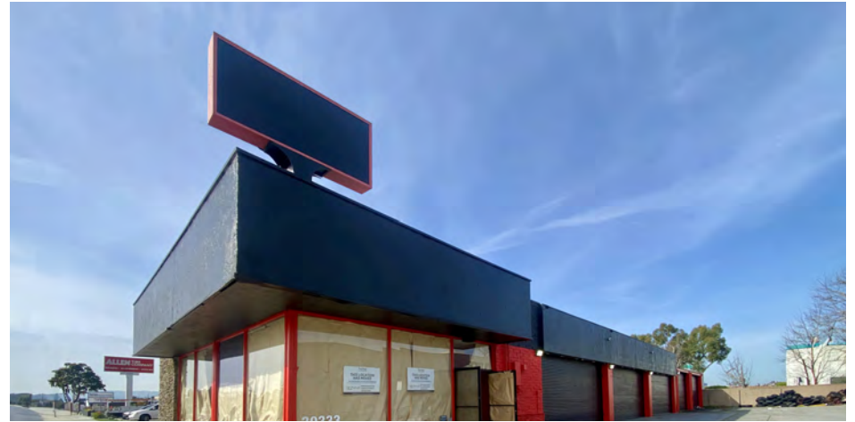
C 20333 Hawthorne Blvd 20333 Hawthorne Blvd, Torrance, CA 90503
