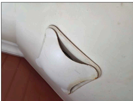
Does not operate - needs to be serviced @ ADU
