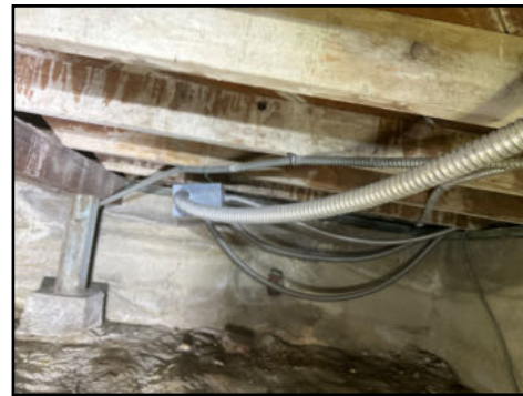
Exposed connections (splices) not properly installed with a junction box - potential hazard - needs to be serviced
