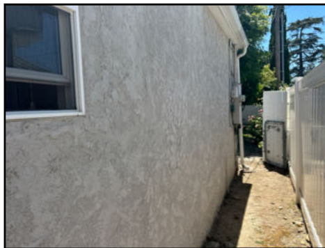
Cold joint cracking present - evidence of past patchwork or addition - check permits and seal joint regularly to ensure against moisture intrusion
