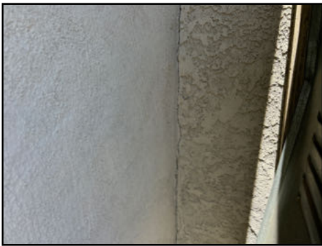
Cold joint cracking present - evidence of past patchwork or addition - check permits and seal joint regularly to ensure against moisture intrusion
