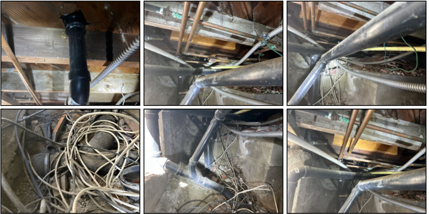
Rubber drain connections present - these are not for long term use - recommend upgrading connections
