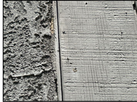
Gaps in siding at joints and around windows/doors - recommend servicing to prevent moisture entry
