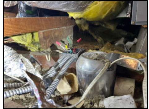
Cover missing at junctions box(es) exposing connections - needs to be serviced
