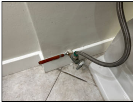
Galvanized water piping present - recommend complete water distribution system evaluation due to age
