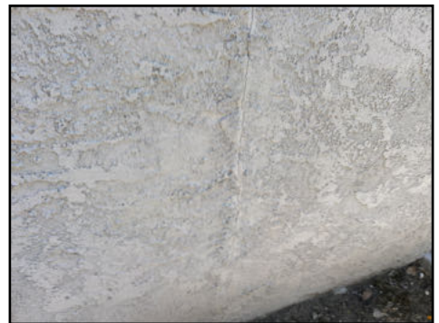
Cold joint cracking present - evidence of past patchwork or addition - check permits and seal joint regularly to ensure against moisture intrusion
