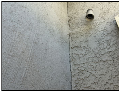
Cold joint cracking present - evidence of past patchwork or addition - check permits and seal joint regularly to ensure against moisture intrusion
