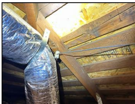
Knob and tube wiring present - old technology, cannot be sure if it has been disconnected - consult an electrician to further evaluate
