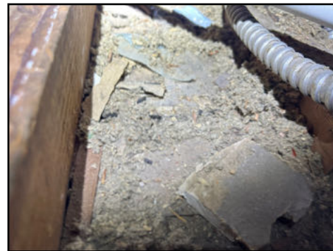
Evidence of rodents/insects/birds/pests - recommend further evaluation by pest services company
