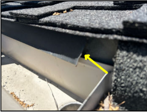
Flashings lifting in areas - needs to be serviced as part of your preventative roof maintenance
