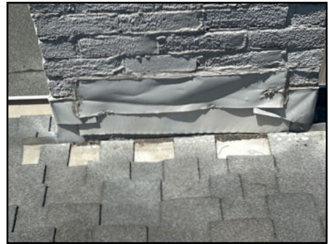
No saddle/cricket at high side of chimney - needs to be serviced
