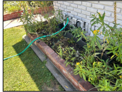
Trees or vegetation too close to structure areas - recommend servicing
