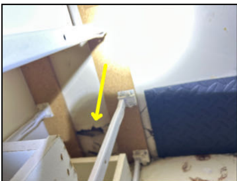
Moisture damage - needs to be serviced - hidden defects may exist
