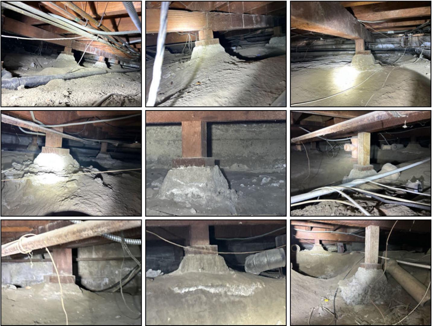
Exposed/undermined post footings - needs to be serviced
