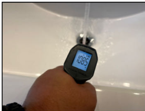
Hot valve did not function properly - needs to be serviced
