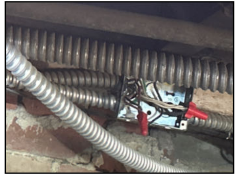
Exposed connections (splices) not properly installed with a junction box - potential hazard - needs to be serviced
