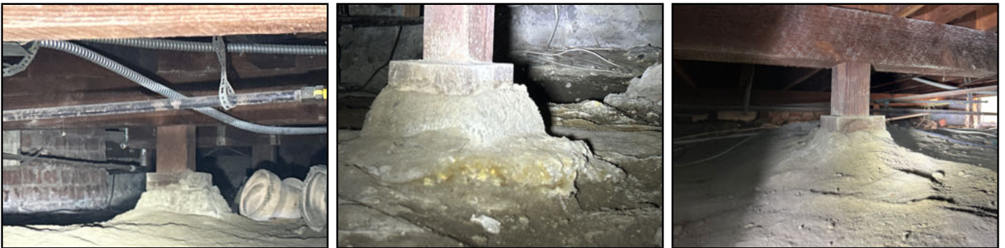
Exposed/undermined post footings - needs to be serviced
