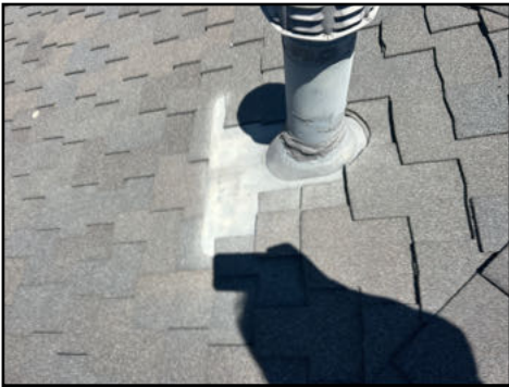
Flashings lifting in areas - needs to be serviced as part of your preventative roof maintenance
