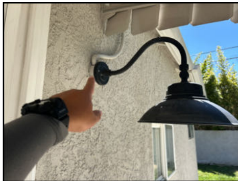
Electrical fixtures need to be caulked/sealed to wall attachments to help prevent moisture entry
