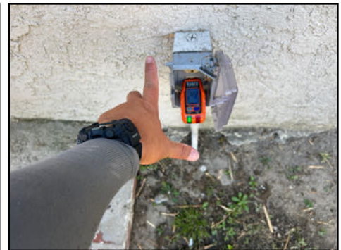
Loose fixture(s) - needs to be serviced
