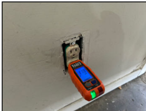
Outlet cover missing - needs to be serviced
