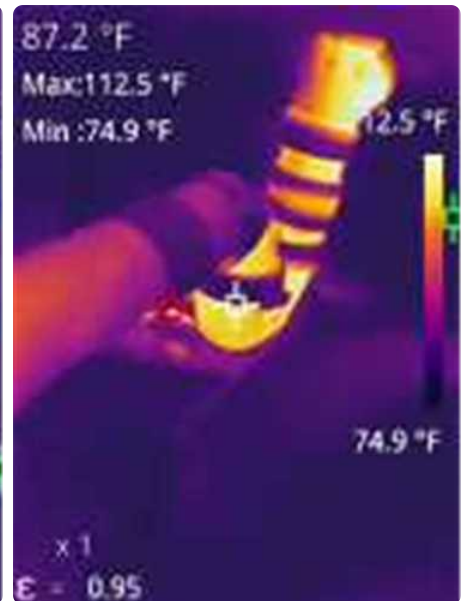
No leaks detected under sinks
