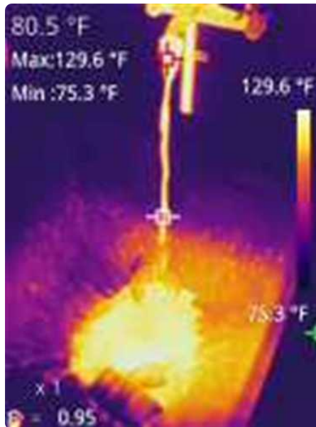
Hot water noted in home
