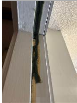
Missing air tight seals - needs to be serviced
