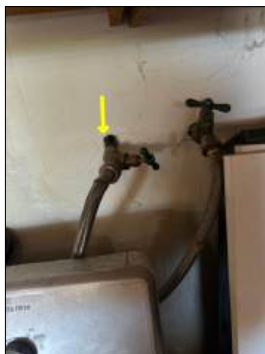
Holes present - needs to be serviced to retain integrity of fire separation
