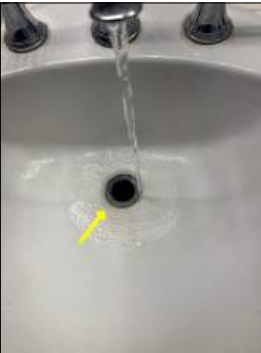
Drain stopper missing - needs to be serviced
