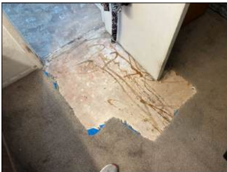
Torn/frayed carpet - typical for age of materials, signs of wear
