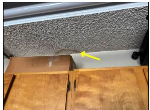
Stains present - tested dry at time of inspection - monitor for future moisture
