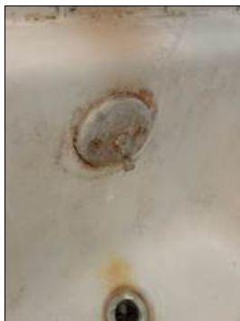
Drain stopper missing - needs to be serviced
