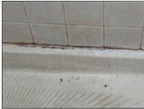
Grout/caulking is dirty or stained - recommend cleaning and drying all surfaces that may accumulate moisture
