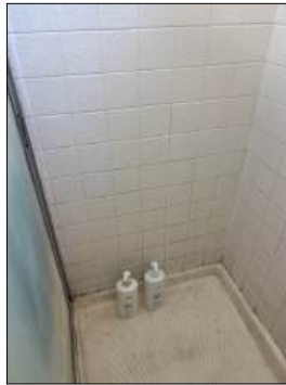
Grout/caulking is dirty or stained - recommend cleaning and drying all surfaces that may accumulate moisture
