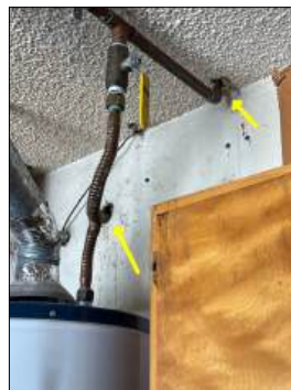
Holes present - needs to be serviced to retain integrity of fire separation
