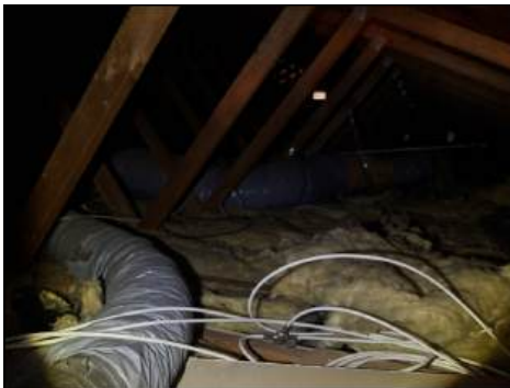
Outer wrap damaged - recommend servicing
