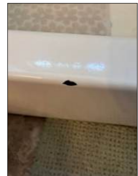
Damaged/rusted/chipped/cracked areas more than typical - needs to be serviced
