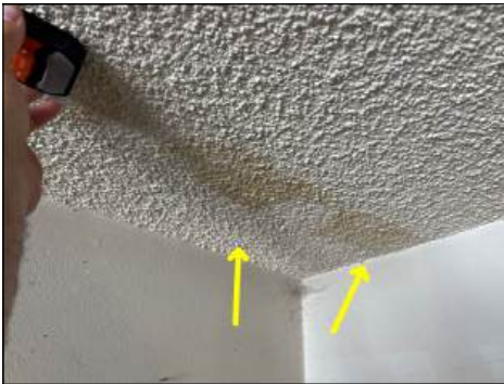
Stains present - tested dry at time of inspection - monitor for future moisture
