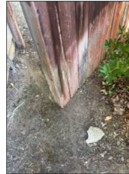
Gate is sagging - recommend servicing
