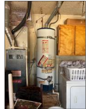
Holes present - needs to be serviced to retain integrity of fire separation
