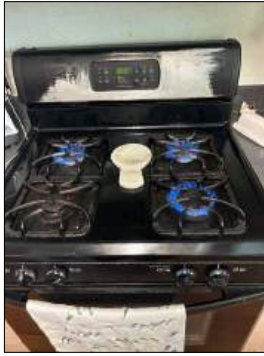
Left front element/burner not operating - needs to be serviced
