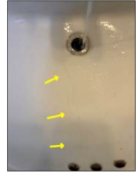
Surface cracking present in sink - signs of age/wear
