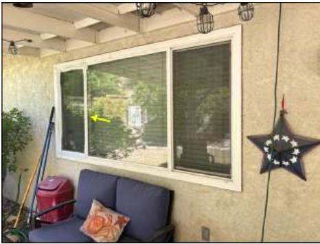
Torn/bent/worn screens - needs maintenance/repair
