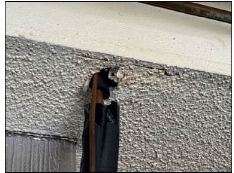
Holes present - needs to be serviced to retain integrity of fire separation
