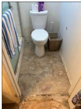
Missing flooring transition(s) - needs to be serviced
