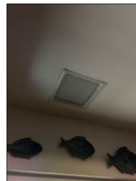
Some bulbs defective/missing/light(s) did not function - check bulbs/consult electrician to further evaluate
