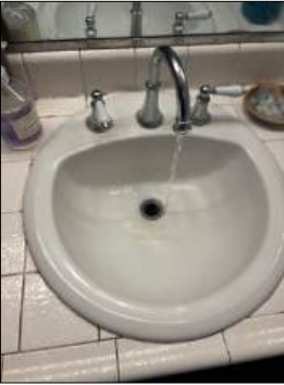
Drain stopper missing - needs to be serviced
