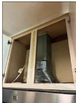
Worn/dirty filters, recommend cleaning or replacing
