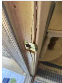
Damaged jamb - needs to be serviced
