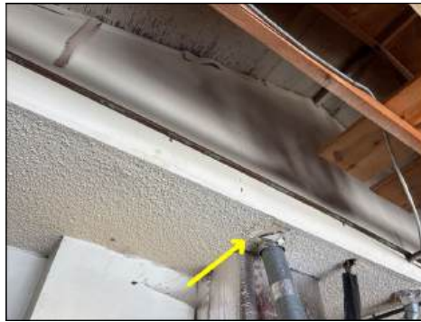
Holes present - needs to be serviced to retain integrity of fire separation
