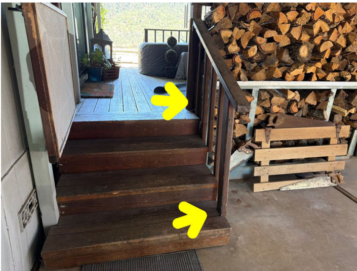
One or more handrails are not secure and should be serviced for optimal safety.
