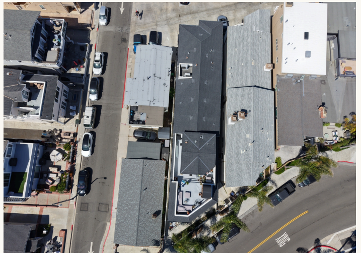
Top-down footprint — rooftop deck, two roof systems visible.
