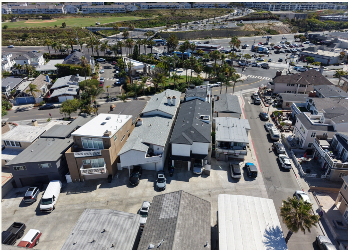
Overhead 3/4 view — Unit A (3-story) and Unit B (2-story).
