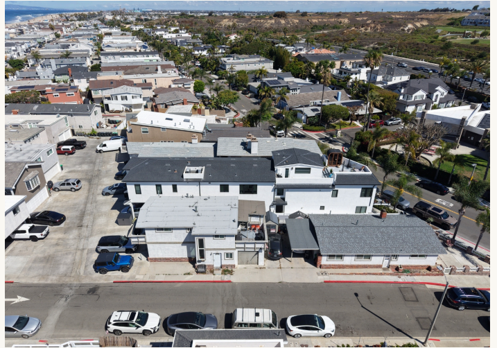
Rear elevation — covered parking and dual-structure layout.
