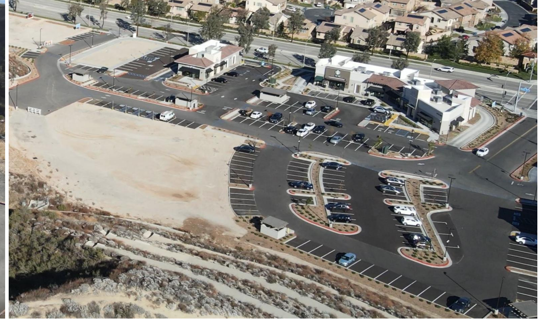
AERIAL FROM HILLSIDE LOOKING DOWN INTO COPPER HILL PLAZA RETAIL
