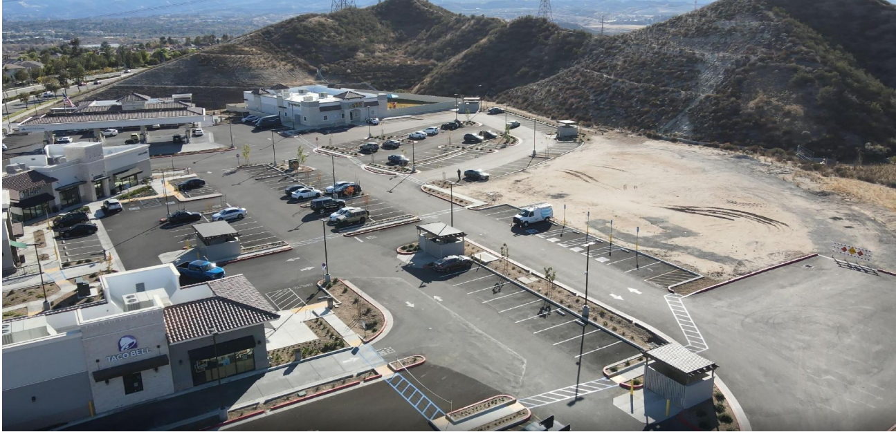
AERIAL OF THE DEVELOPMENT PAD WITHIN COPPER HILL PLAZA RETAIL
