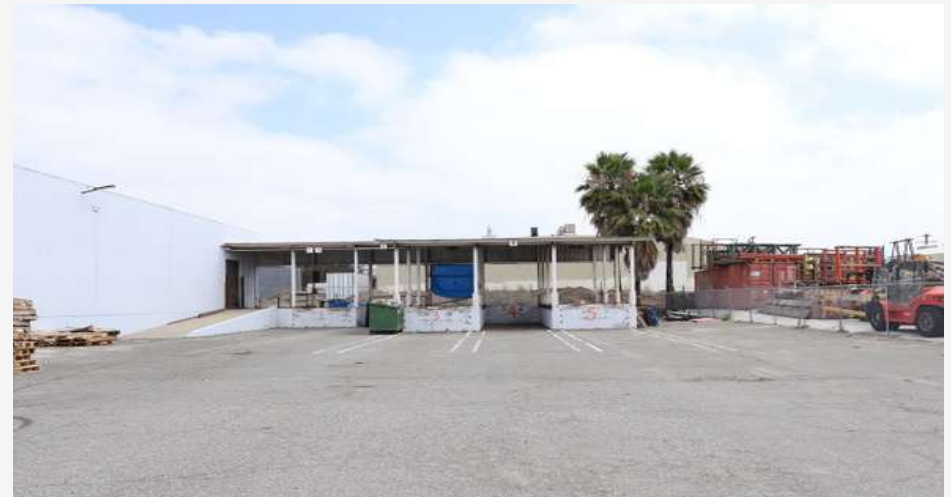
Dock High Loading & Ramp
