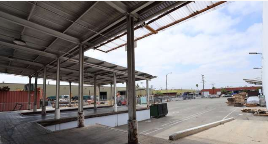
Dock High Loading & Ramp
