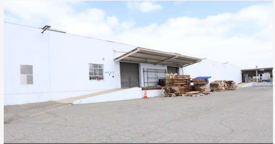
Dock High Loading & Ramp
