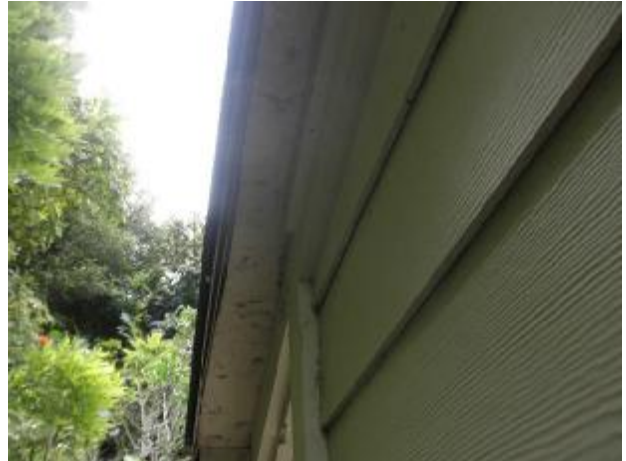
OSB plywood used at parts of the exterior eaves.
