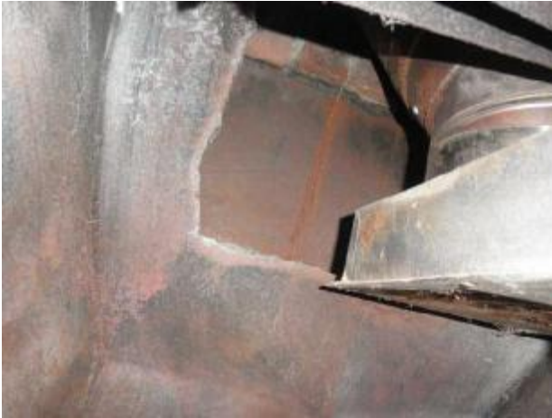
Fireplace has been cut open for a wood stove conversion.
