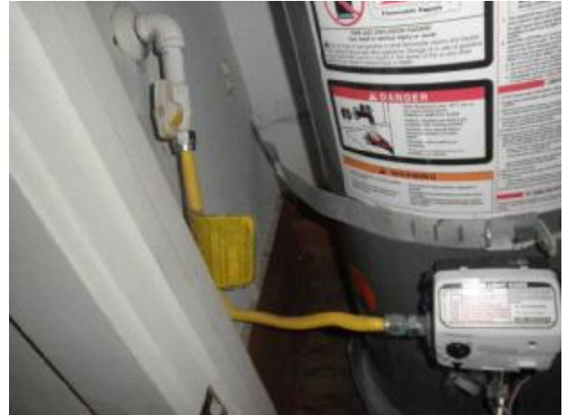
Missing sediment trap at the gas line connection to the water heater.
