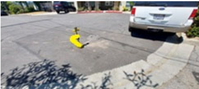
Additional section of fiberglass lined pipe. Depth 4'.
