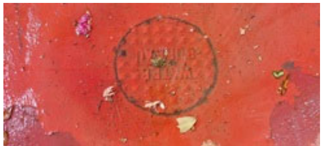
Third inspection through this main cleanout.
