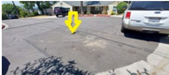
Connection to city sewer line. Depth about 10'.
