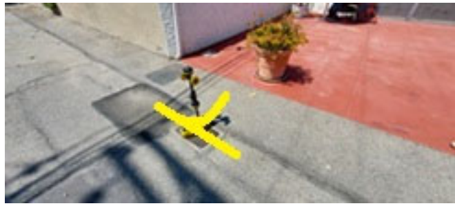
Path of pipe. Possible side line connection from neighbor. Depth 2 ½'.
