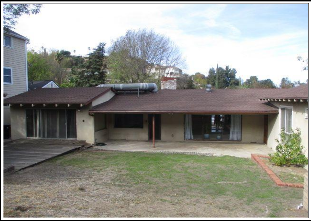
REAR OF SUBJECT PROPERTY
