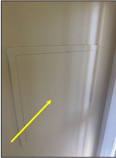
Access for faucet shut offs in the laundry room
