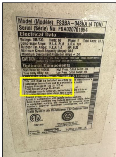
Monitor R22 Refrigerant: The AC unit uses R-22 refrigerant
