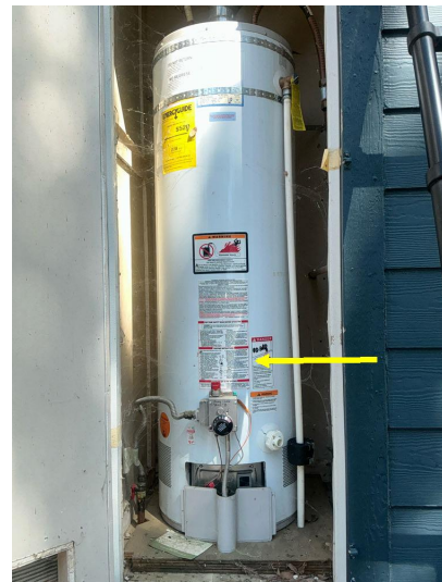
The water heater is not correctly secured, and needs to be seismically strapped and braced in accordance with local standards.
