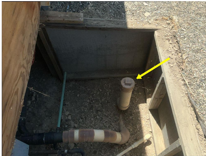
A clean-out is located at the rear.
