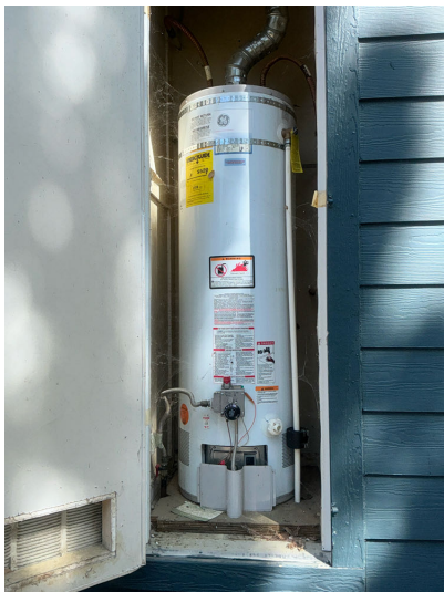
Hot water is provided by a 40 gallon gas water heater that is located in the exterior closet.
