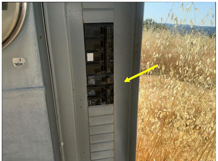
Various circuits are not labeled, which is recommended.
