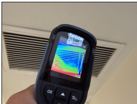
Temperature at Air Return
