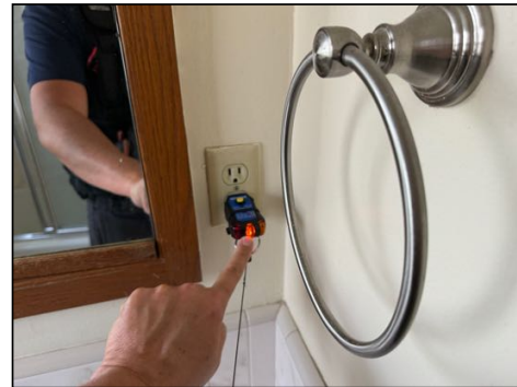
Three prong outlet(s) not grounded - needs to be serviced - both
