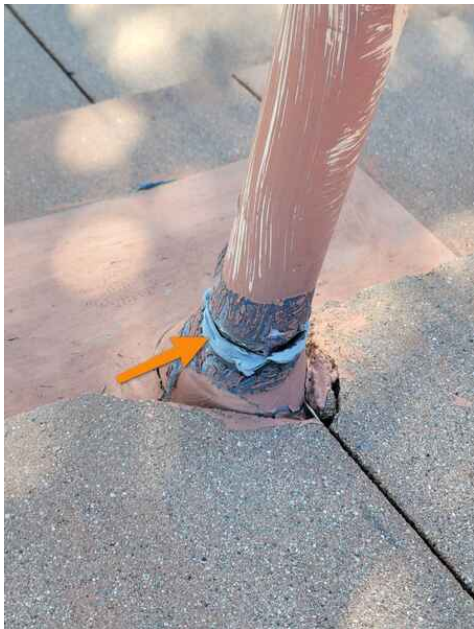
all pipe penetrarions' sealant is cracked
