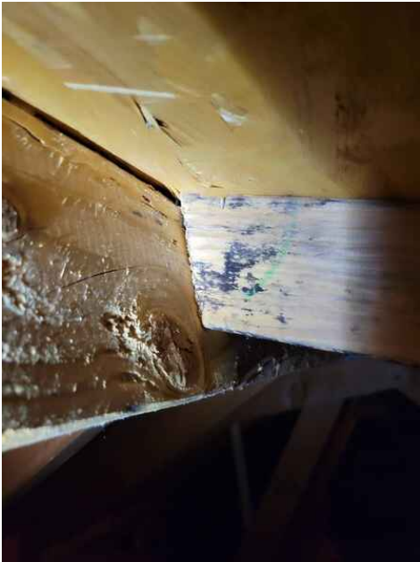
possibly typical lumber mold but we recommend testing this area in the attic when other areas are tested
