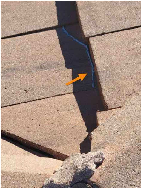
improper repair to broken tile
