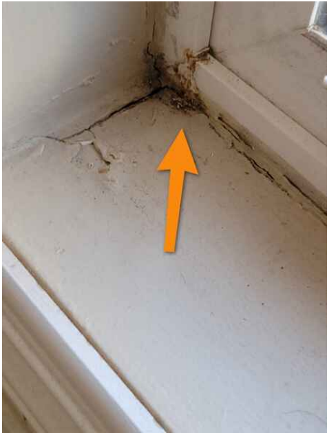
moisture/mold damage
