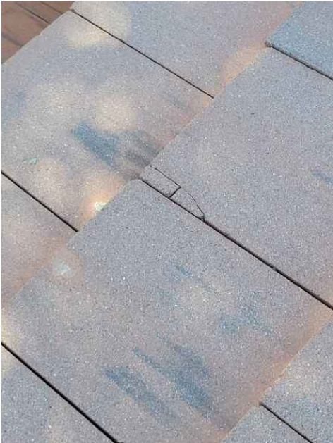
improper repair to broken tile
