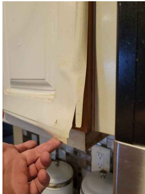
heat damage from improperly vented cooktop
