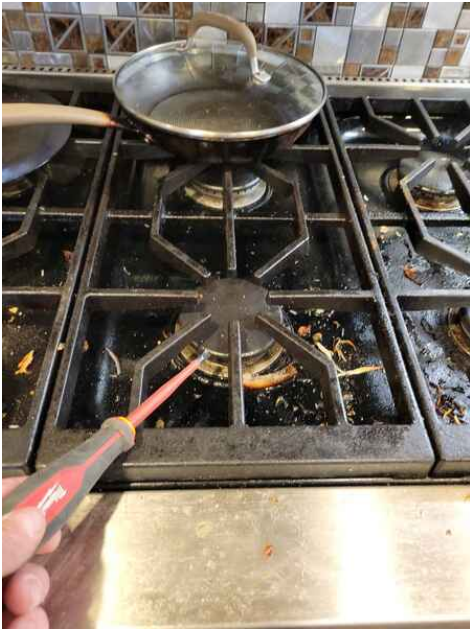
burner ignitor failure
