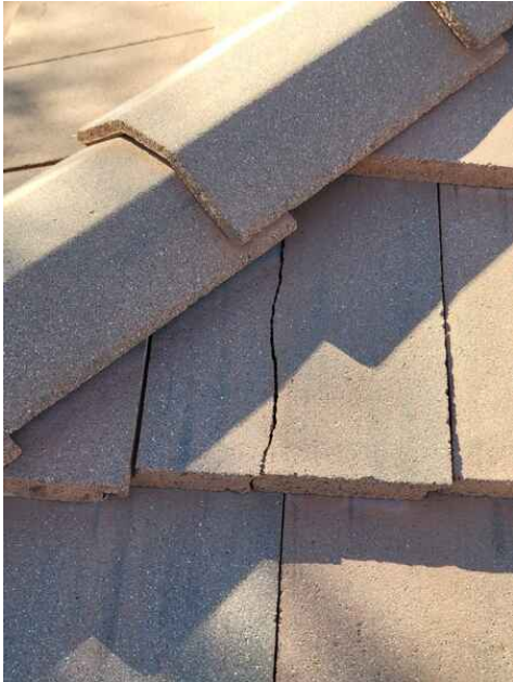
improper repair to broken tile
