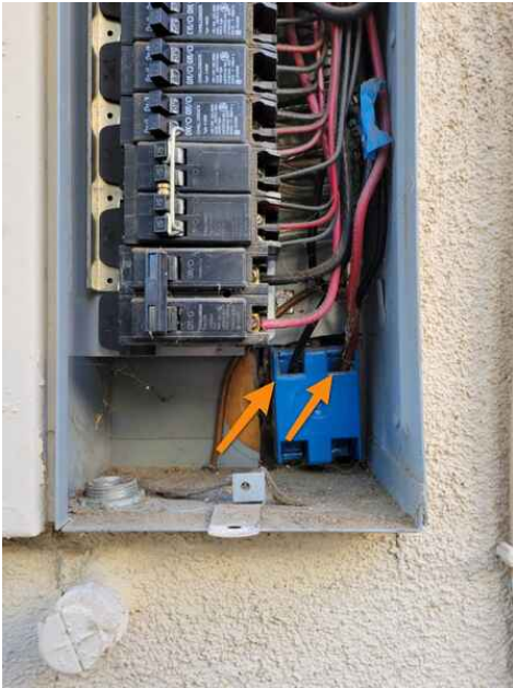
this box is not rated for a 240-volt outlet.
