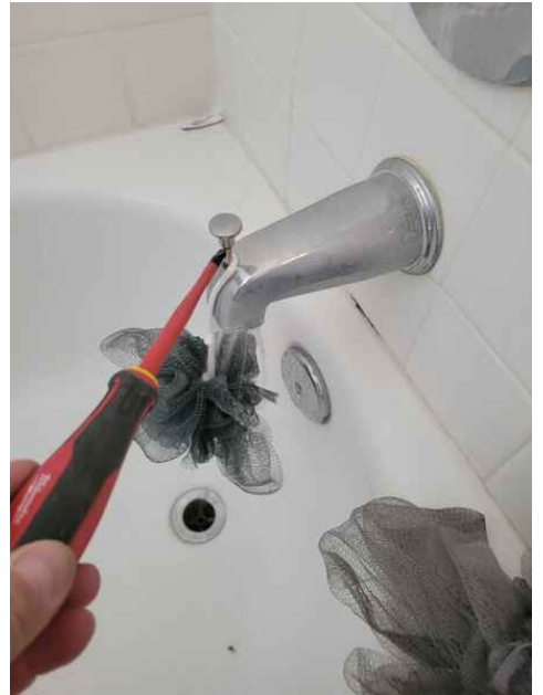
tub spouts all stuck in shower position
