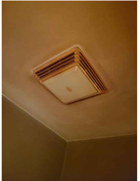
dripping from ceiling and running down walls exhaust fans are beyond repair/cleaning
