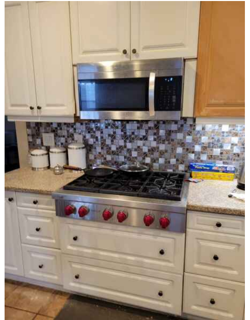
a minimum of a 36-inch-wide hood is required for this cooktop
