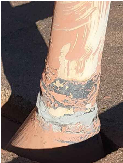
all pipe penetrarions' sealant is cracked
