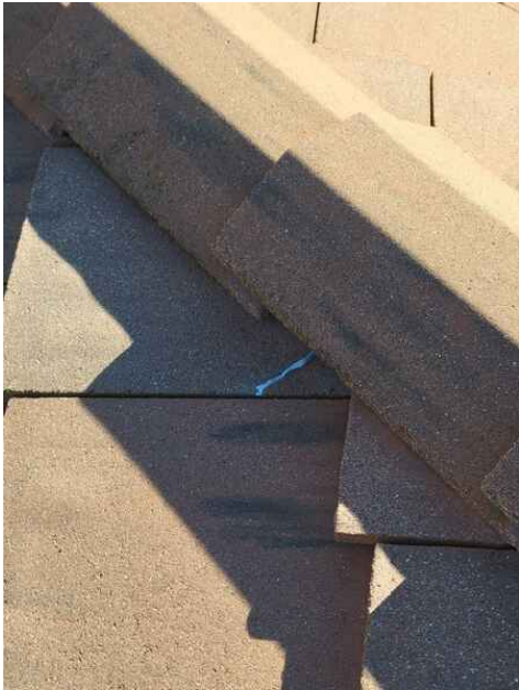
improper repair to broken tile
