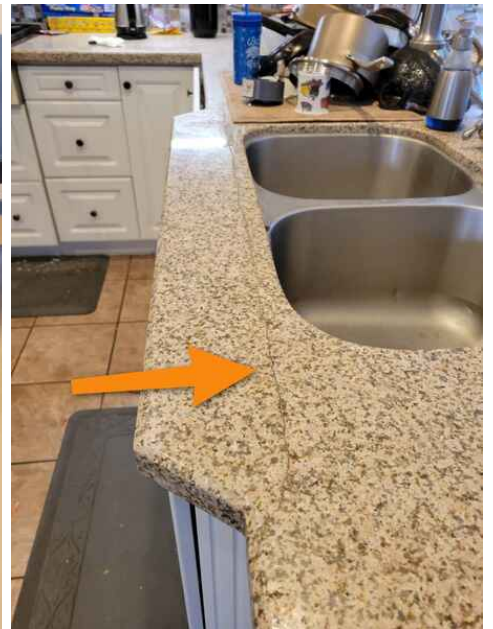
countertop is cracked and previous repair attempt has failed
