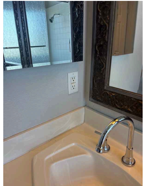
Master Bathroom is connected to 2nd Floor guest bathroom
