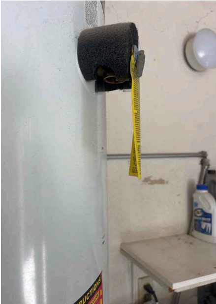
General: Location Garage
