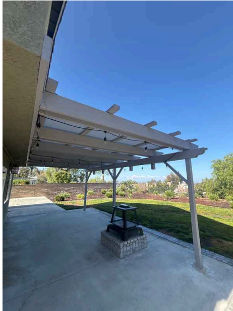
Fences, Gates: Fence, Gate Condition Serviceable
