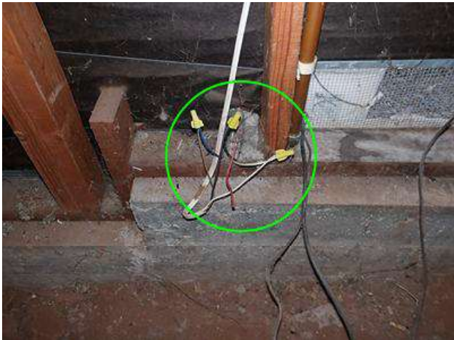
Photo 38-1 Crawl space West side
