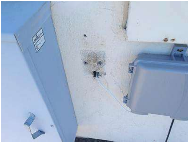
Photo 15-1 NE corner garage
