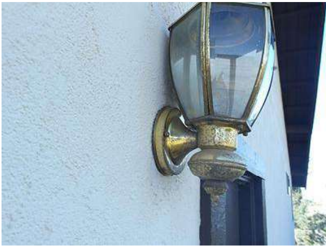
Photo 43-3 North side garage
