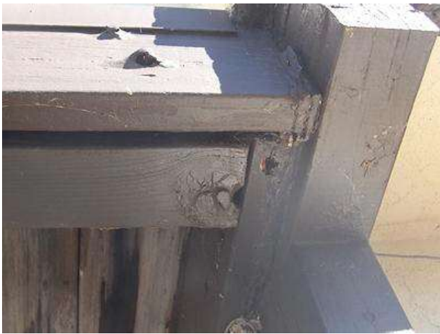
Photo 5-5 South end deck
