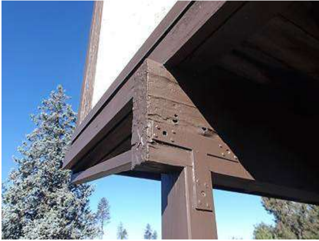
Photo 5-3 South end deck
