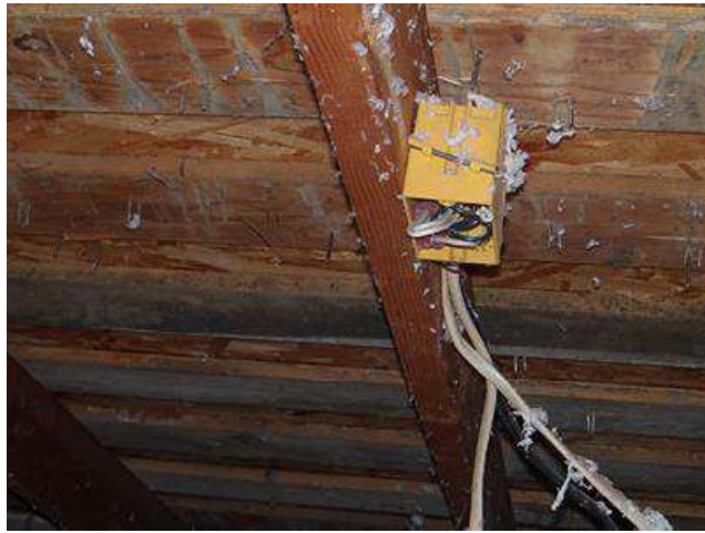
Photo 42-2 Attic above master bathroom
