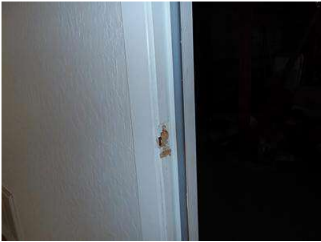
Photo 18-1 Crawl space entry door
