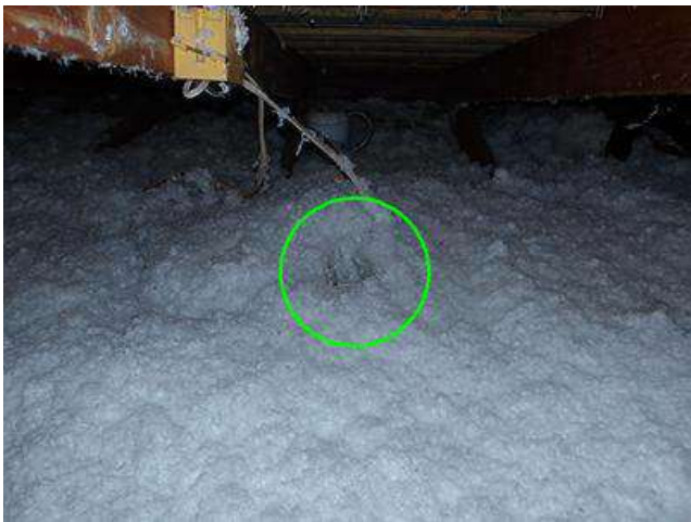
Photo 21-3 Master bathroom exhaust fan termination
