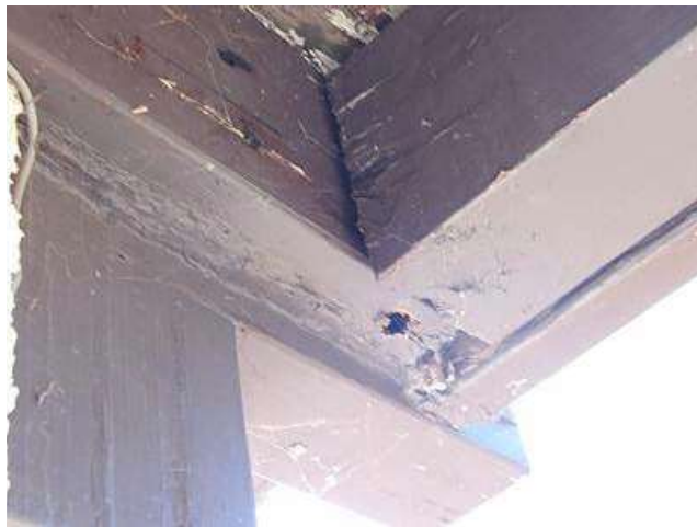
Photo 5-8 South end deck
