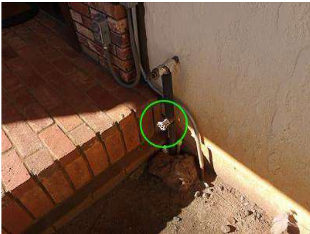
Photo 54-1 Water shut-off, East side
