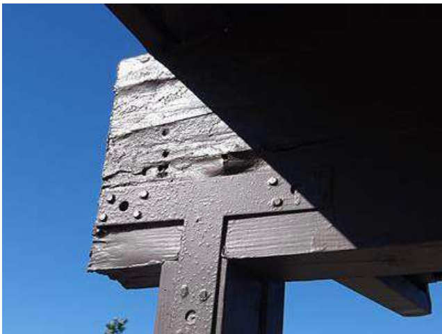
Photo 5-7 South end deck
