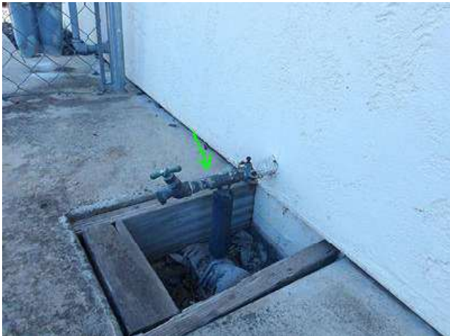
Photo 51-1 North side garage
