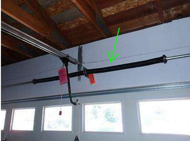
Photo 27-1 North vehicle door spring
