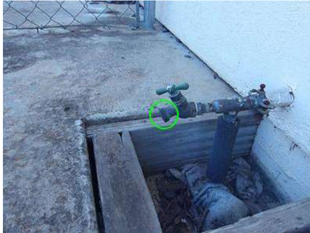
Photo 53-2 North side garage
