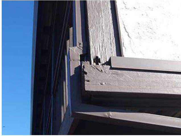
Photo 5-4 South end deck
