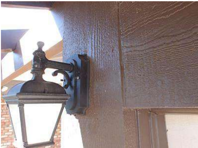
Photo 43-1 SE corner garage
