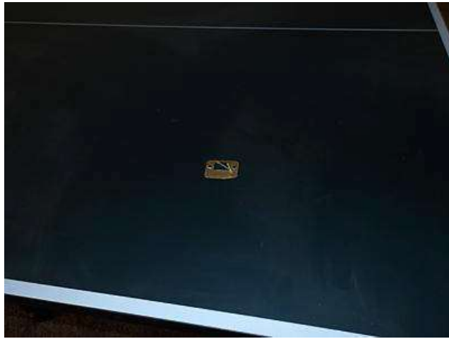
Photo 18-2 Crawl space entry door (uninstalled hardware)
