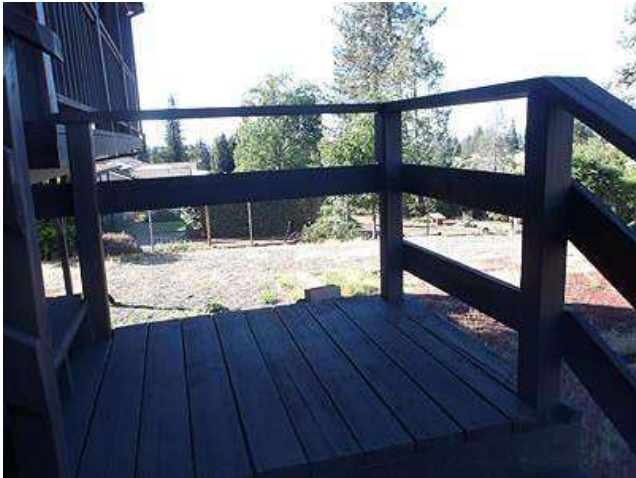
Photo 2-1 Deck stair landing
