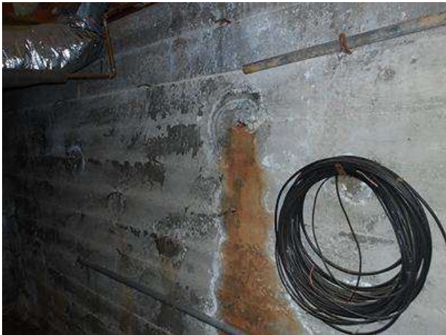
Photo 19-1 Crawl space East wall
