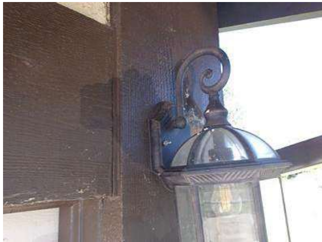
Photo 43-2 NE corner garage
