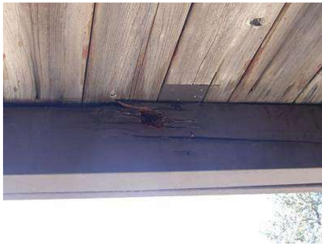
Photo 5-6 South end deck
