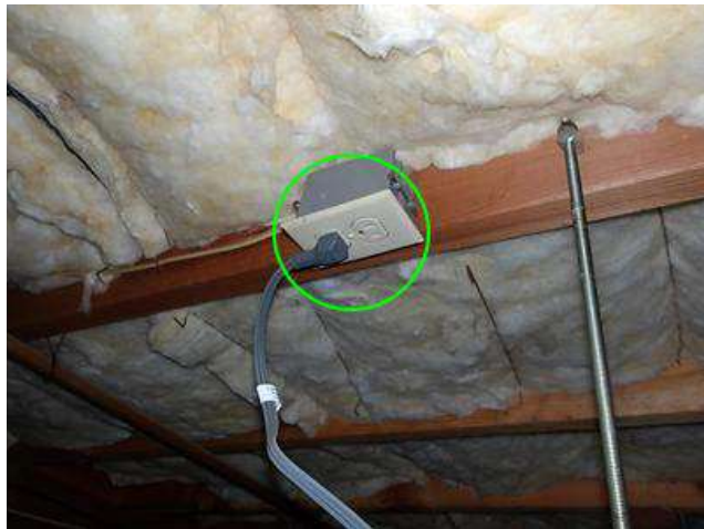
Photo 33-2 Crawl space above furnace
