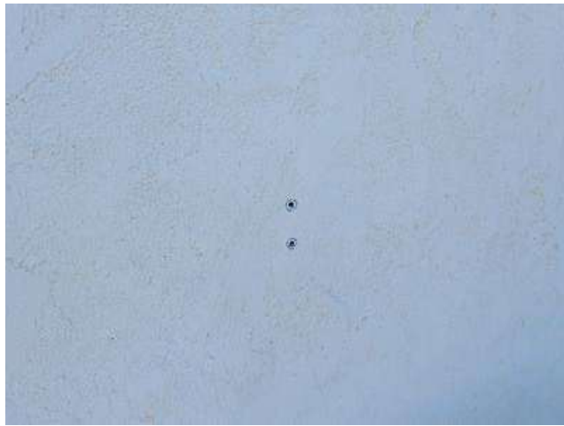
Photo 15-2 North side garage
