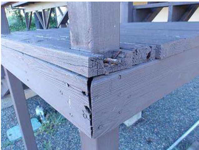
Photo 5-1 Deck stair landing
