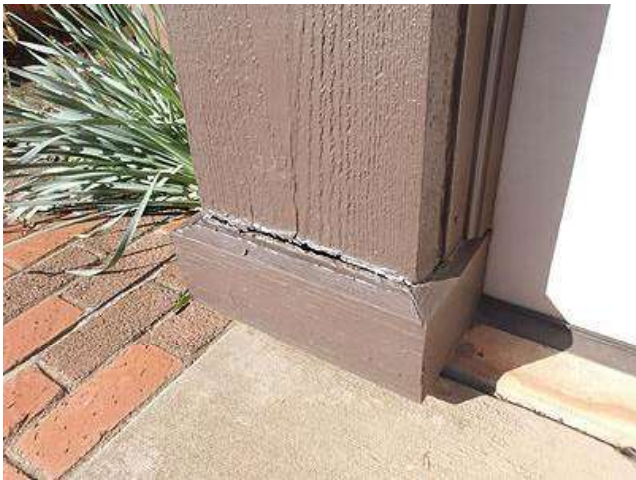
Photo 13-1 SE corner garage
