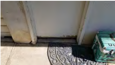
Stucco Intersection with Door Frame
