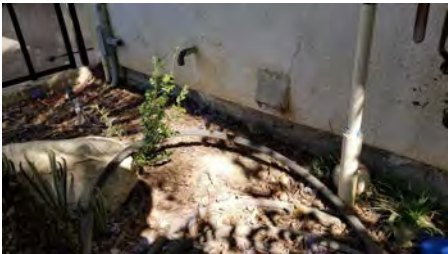
Stucco Termination at Grade
