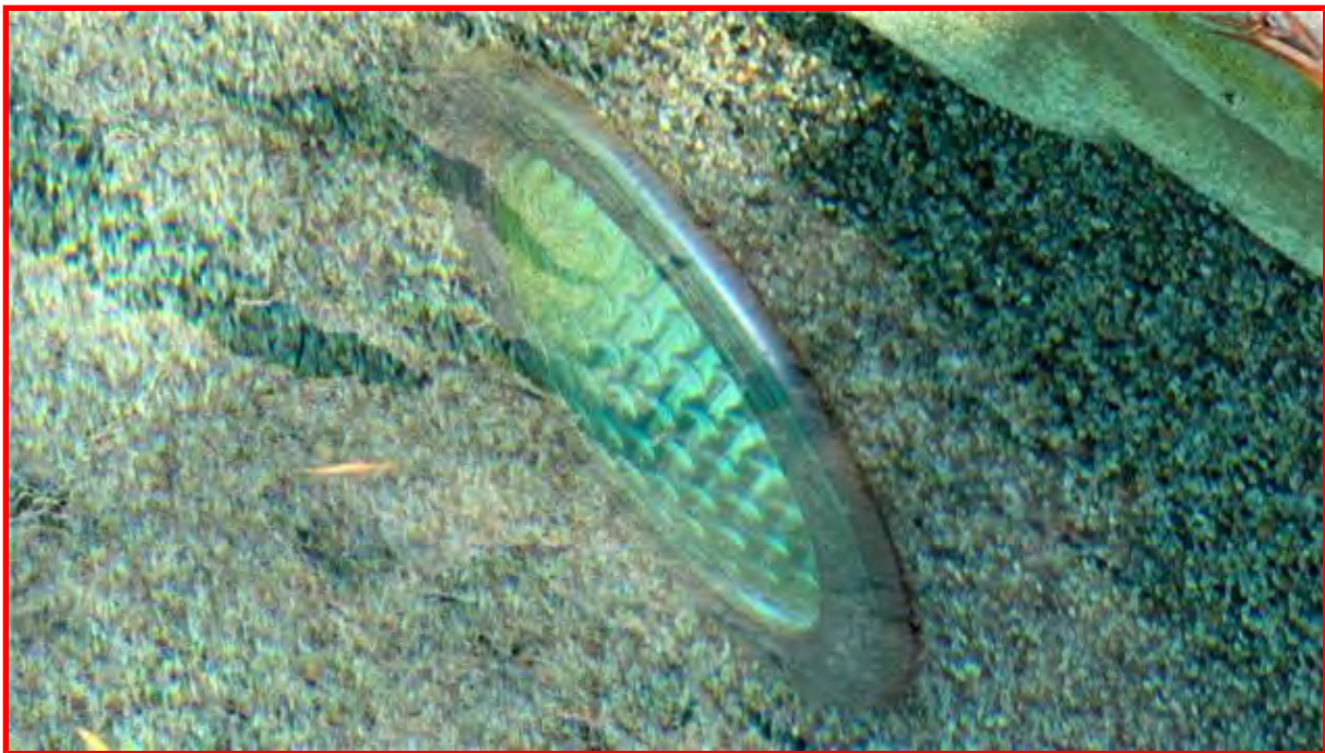
Pool / Spa Light Not Functioning
