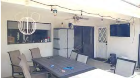
Rear Door and Windows Protected by Covered Porch
