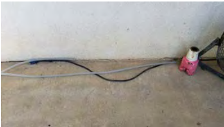
Stucco Termination at Concrete Porch
