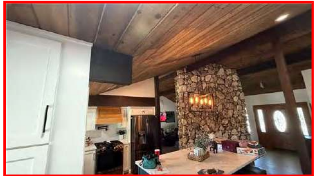
Wall Beam Removed in Kitchen Area
