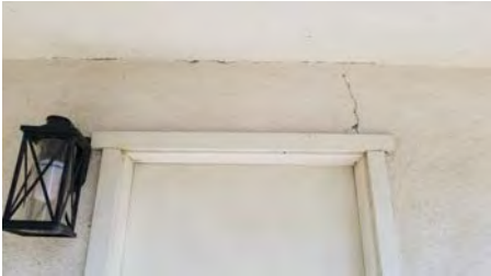
Stucco Intersection with Door Frame
