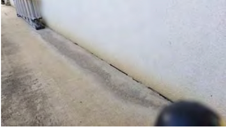
Stucco Termination at Concrete Porch
