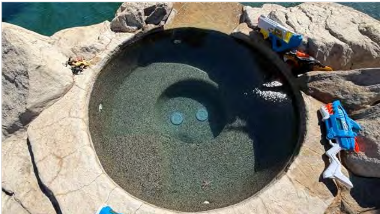
Spa Drain Covers
