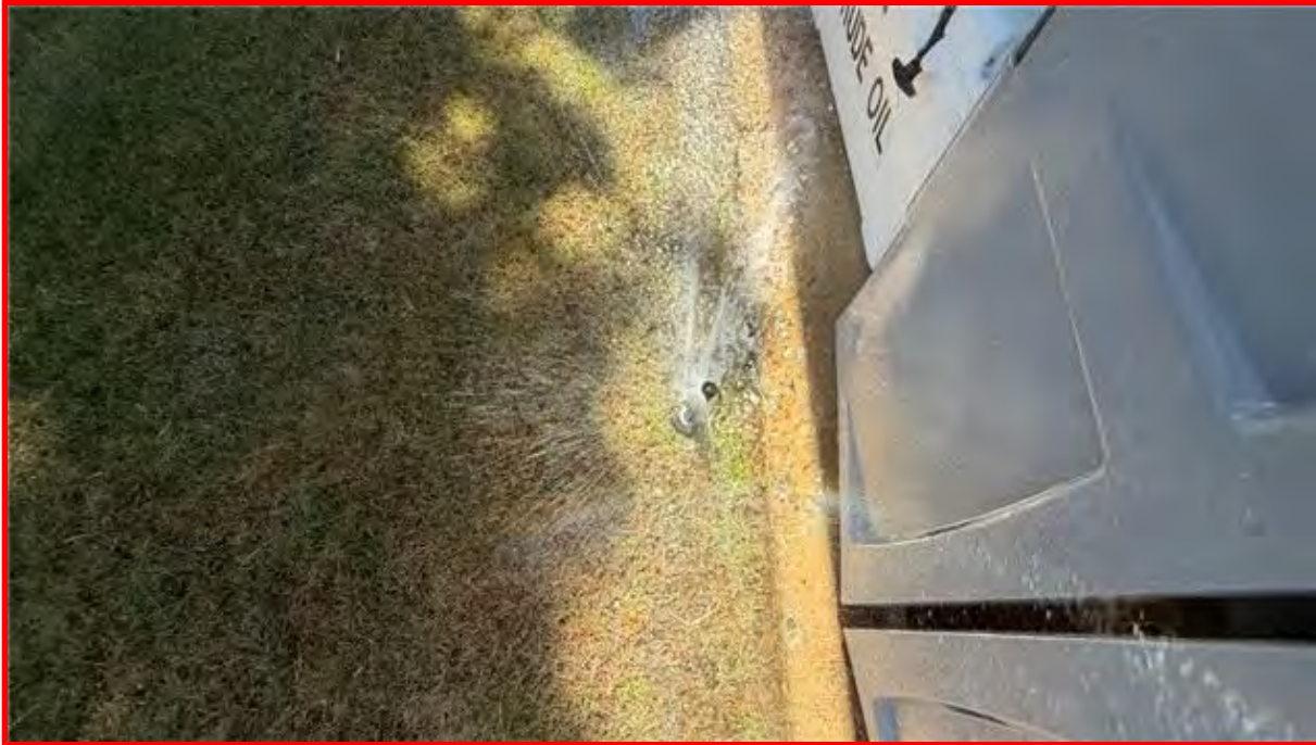
Damaged Rear Small Yard Sprinkler
