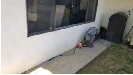
Stucco Termination at Concrete Porch
