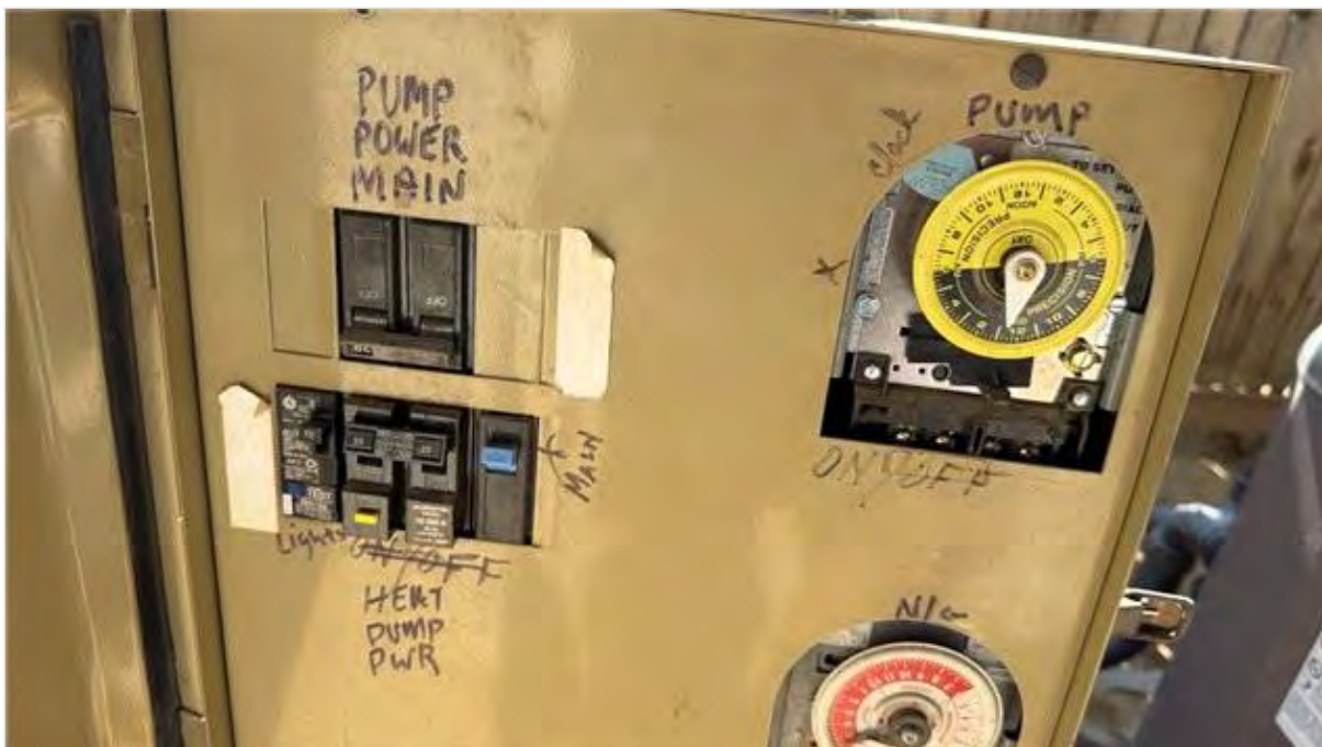
Panel Timer and Breakers
