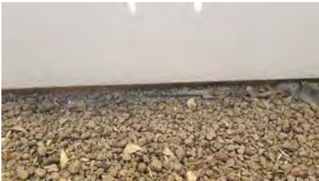
Stucco Termination at Grade
