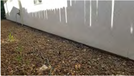
Stucco Termination at Grade
