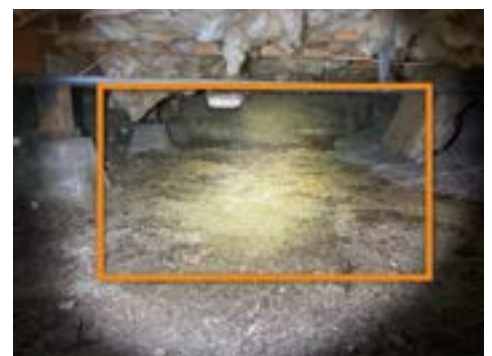
Front Right Crawlspace
