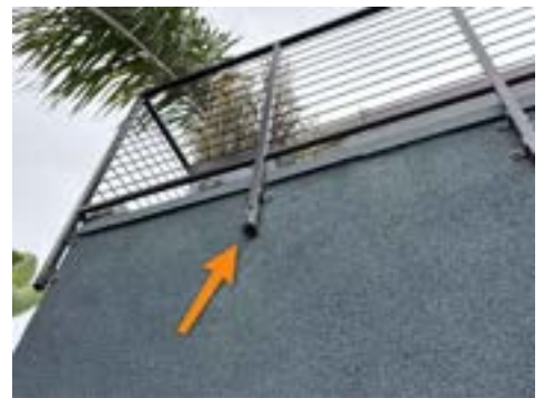
Front Right Exterior Balcony
