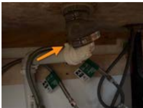
Master Bathroom Left Sink
