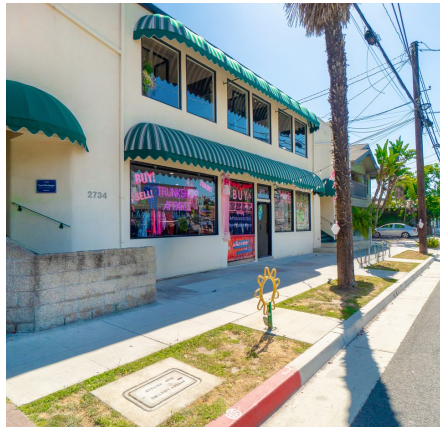
Building entry — Suite 7 street access
