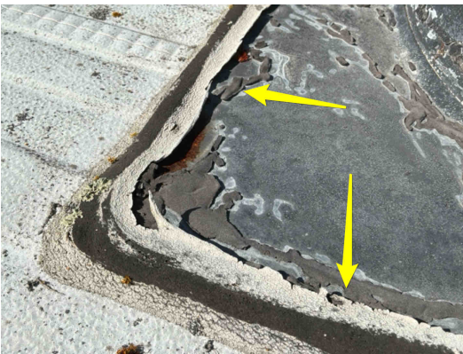
Deteriorated sealant around the fireplace chimney roof flashing
