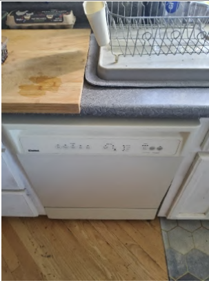
Dishwasher is not properly fastened, recommend repair
