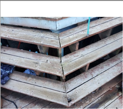
Damaged tread members, recommend replacing
