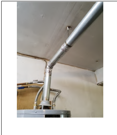
Vent cap loose, recommend repair
