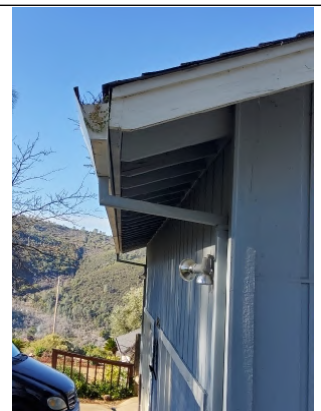
Gutter is full of debri and rusting, recommend cleaning
