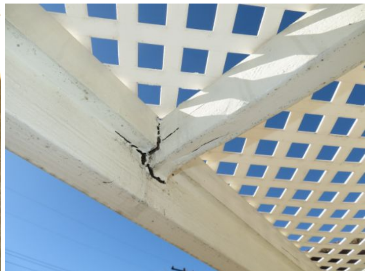
deteriorated wood
