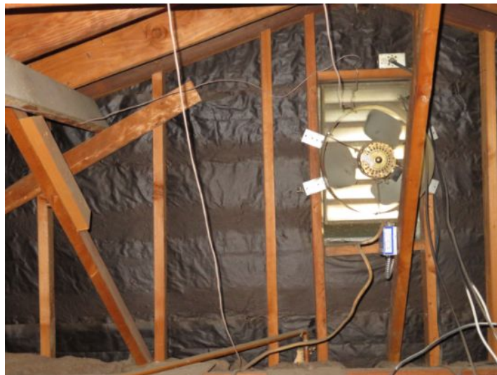
attic fan present, not tested by the inspector
