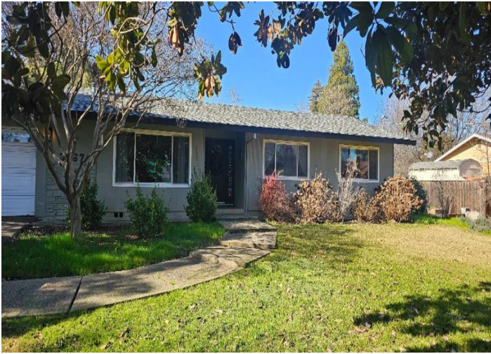
Front of the structure.
