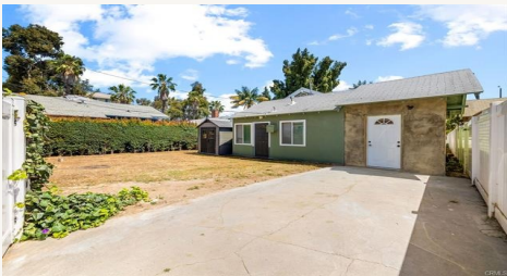
Rear unit, private driveway, and open lot
