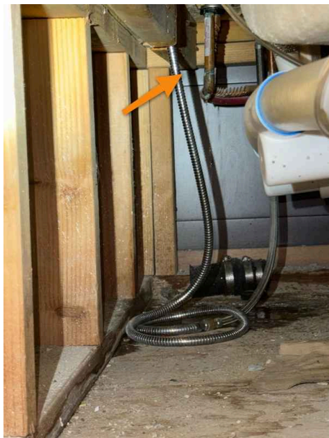
2nd Floor Primary Bathroom
