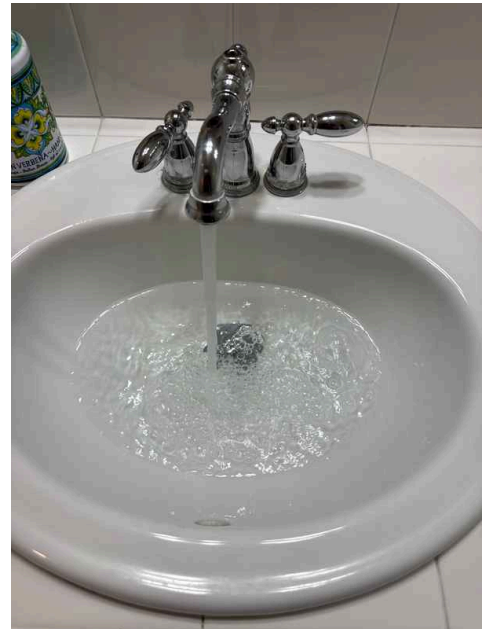
2nd Floor Jack & Jill Bathroom
