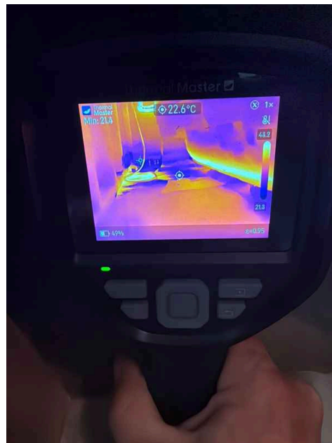
2nd Floor Primary Bathroom
