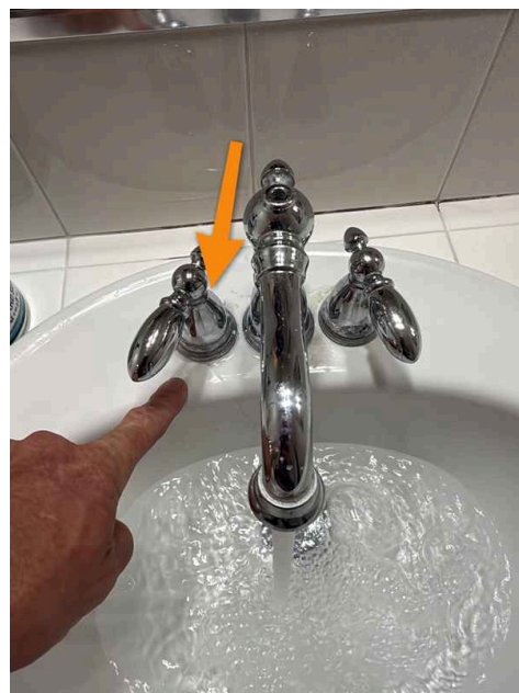
2nd Floor Jack & Jill Bathroom
