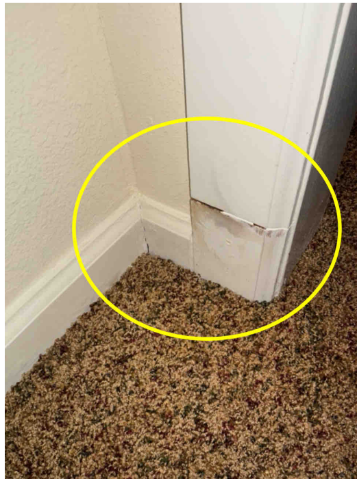
Example. Inside the closet
