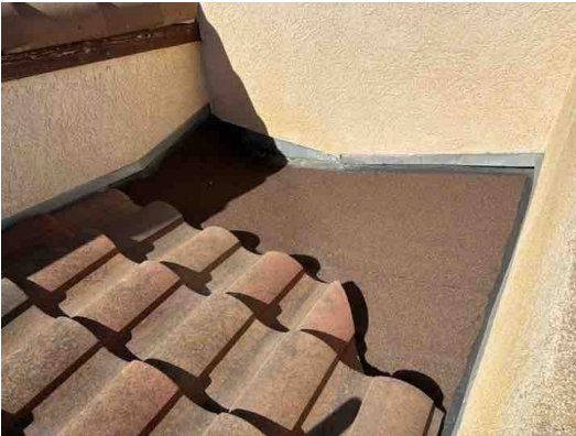
55: Roof was walked
