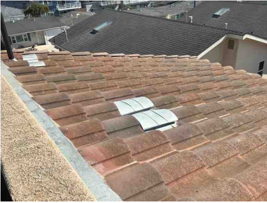
54: Rolled Asphalt Composition Roof Crickets
