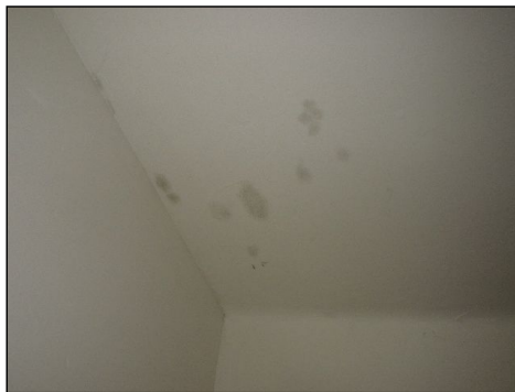
Microbial growth/irregular staining present- in closet in ADU
