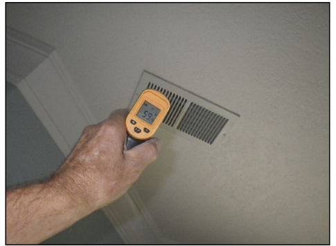
A/C Temperature at Registers: 50 - 57 degrees main structure, 60 degrees ADU
