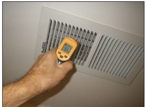
A/C Temperature at Registers: 50 - 57 degrees main structure, 56 - 60 degrees ADU
