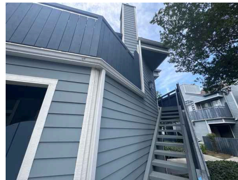
Foundation: Material Concrete, Slab on Grade
