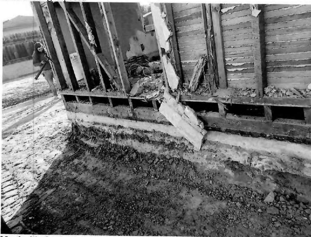
North side footing exposed
