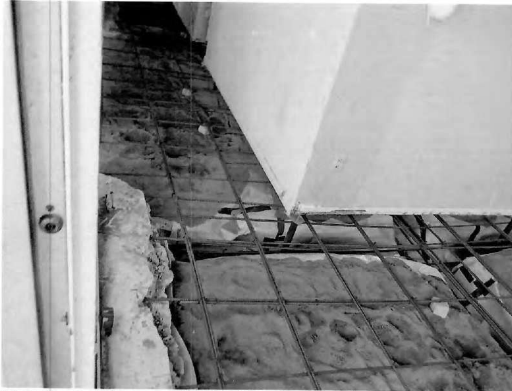
Photo showing pipes supporting interior wall of a residence
