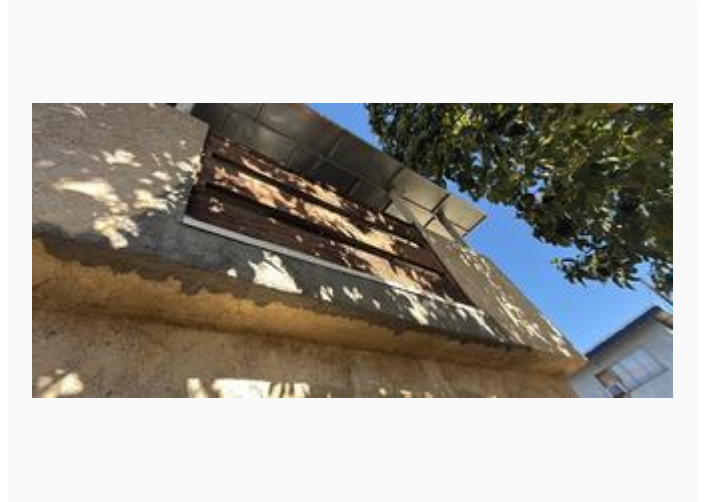
Stucco has been repaired recently
