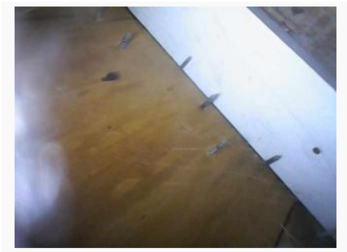
Structural integrity, good with no signs of water or damage
