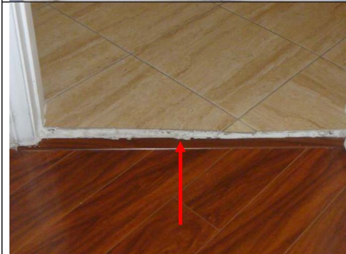
Step along the office entry doorway.
