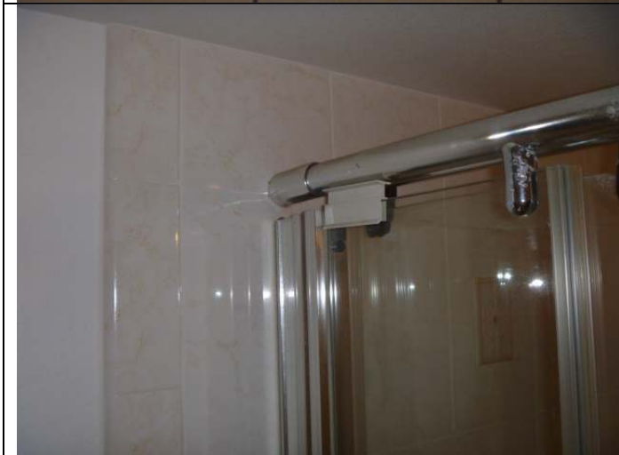
Downstairs bathroom shower. Note: The tiles backing type was not determined.
