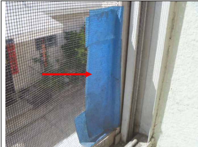
West bedroom window screen repair.
