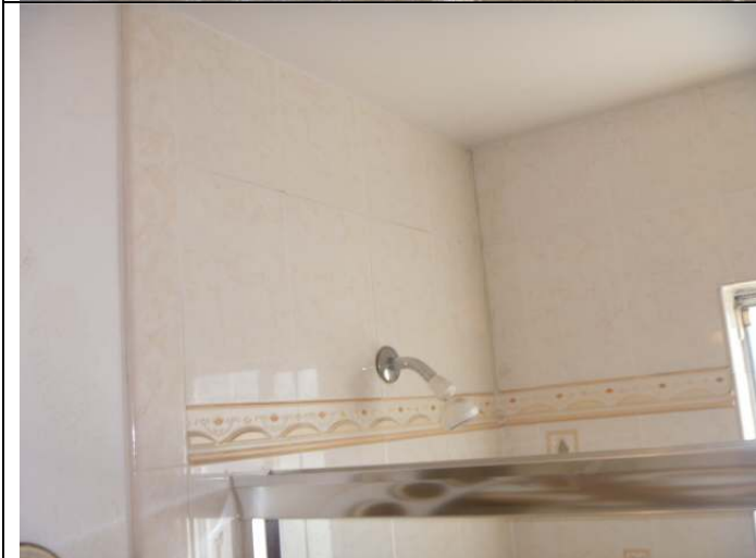
Full bathroom shower/tub. Note: The tiles backing type was not determined.
