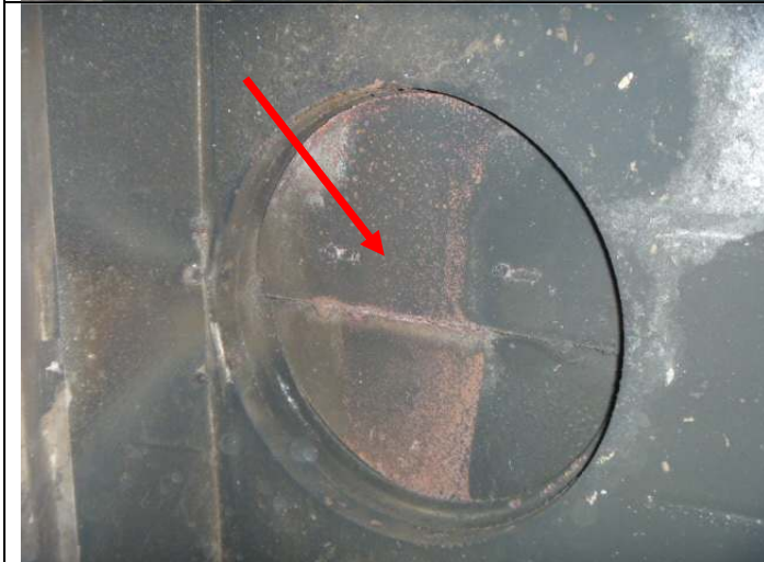
Fireplace damper in the closed position.
