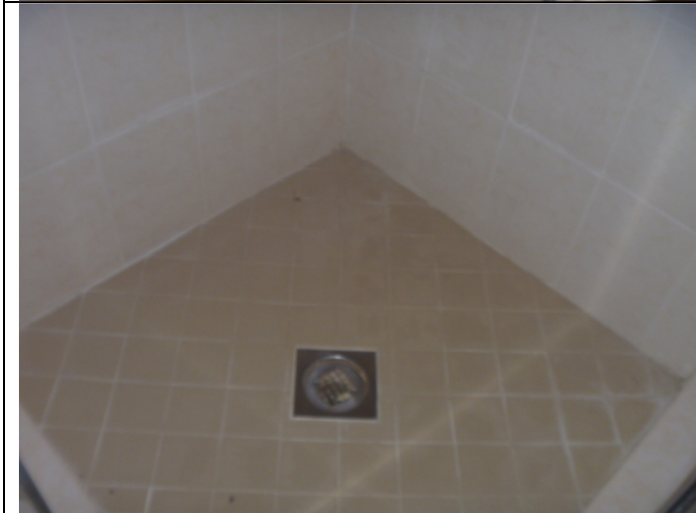
Upstairs 3/4 bathroom shower.
