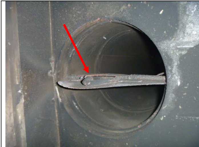
Fireplace damper in the open position.
