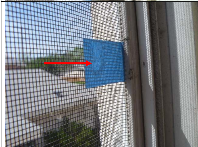
West bedroom window screen repair.
