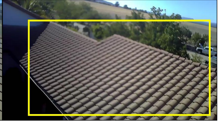
At the time of the inspection the majority of the roof was in good condition.
