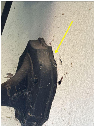
Exterior lighting was installed in a manner that left energized electrical components exposed to moisture intrusion.
