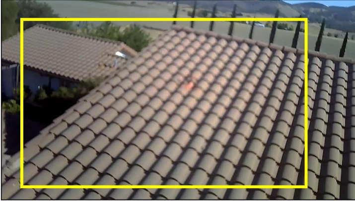
At the time of the inspection the majority of the roof was in good condition.
