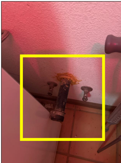
Plumbing in place if washbasin is desired to be installed
