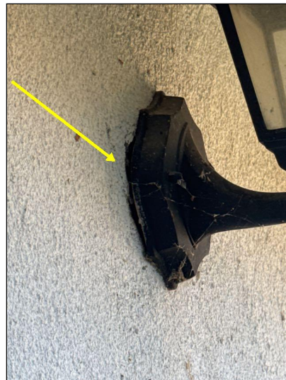
Exterior lighting was installed in a manner that left energized electrical components exposed to moisture intrusion.
