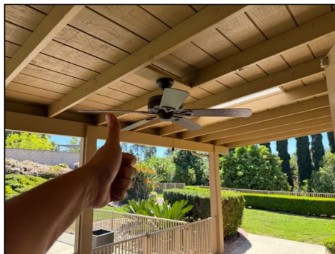
Electrical fixtures need to be caulked/sealed to wall attachments to help prevent moisture entry
