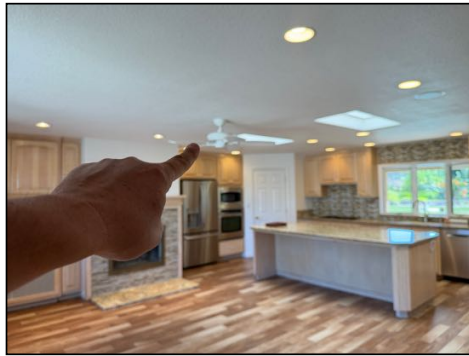
Did not operate - needs to be serviced or further evaluated - kitchen area
