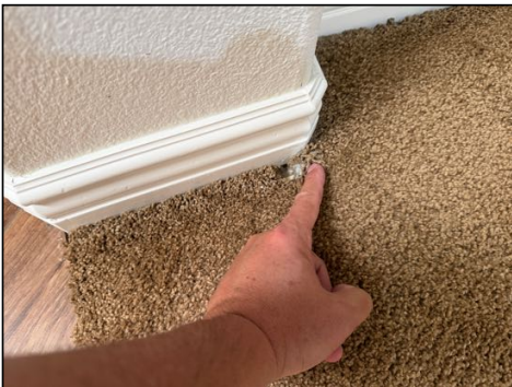
Torn/frayed carpet - typical for age of materials, signs of wear - master
