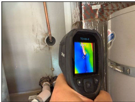
Air leaking at refrigerant or condensate line connection areas - needs to be sealed to prevent air loss - both
