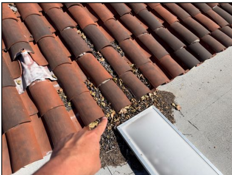
Vegetation on roof - not fully visible for inspection - recommend servicing/cutting back vegetation away roof areas
