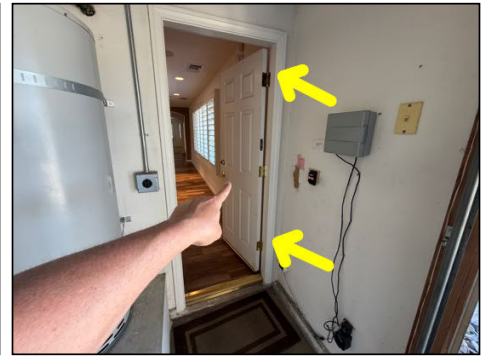
Self-closing device not operating - needs to be serviced
