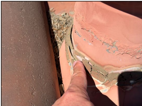
Mastic at vent(s) is weathered and cracked - needs to be serviced and resealed at all penetration points
