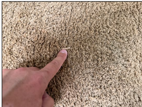
Torn/frayed carpet - typical for age of materials, signs of wear - master
