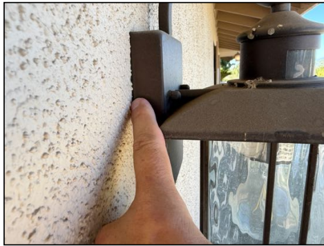
Electrical fixtures need to be caulked/sealed to wall attachments to help prevent moisture entry
