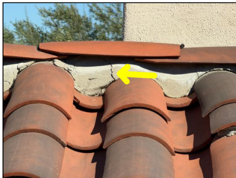
Cracked/chipped tiles/mortar - typical for age/materials - recommend seasonal roof maintenance
