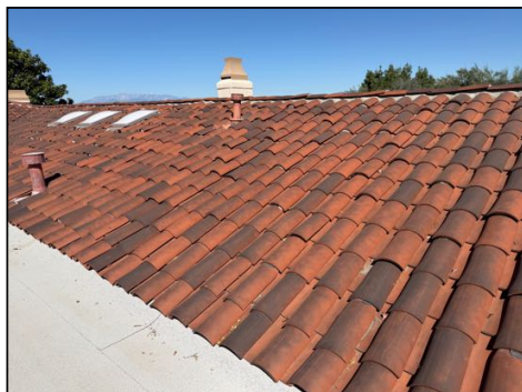
Cracked/chipped tiles/mortar - typical for age/materials - recommend seasonal roof maintenance
