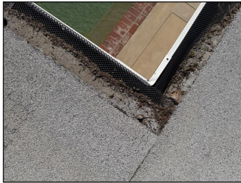
Gutter leaf guards may allow water to bypass - inquire with seller
