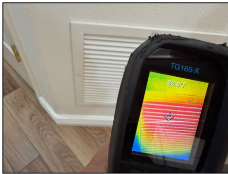
Temperature at Air Return
