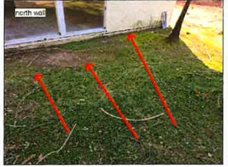
Stained areas show evidence of ponding water or poor drainage – recommend further evaluation
