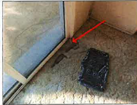
Worn/stained areas near doors - evidence of past moisture entry point - needs to be serviced
