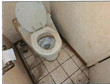
Toilet loose at floor - needs to be serviced
