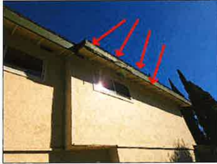
Condensation/moisture damage - needs to be serviced - consult the termite report
