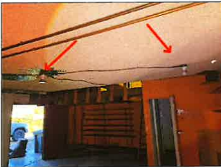
Some bulbs defective/missing/light(s) did not function - check bulbs/consult electrician to further evaluate
