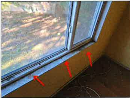
Stains/blisters at sill - tested dry for moisture at the time of the inspection - monitor the areas for moisture intrusion
