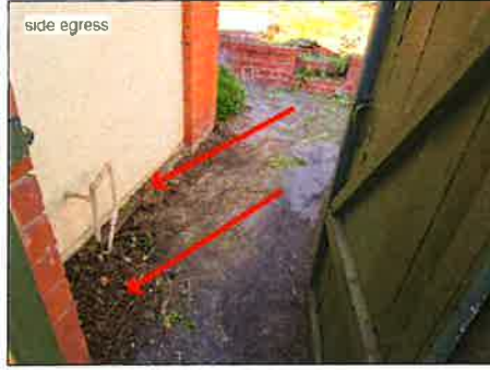
Stained areas show evidence of ponding water or poor drainage – recommend further evaluation
