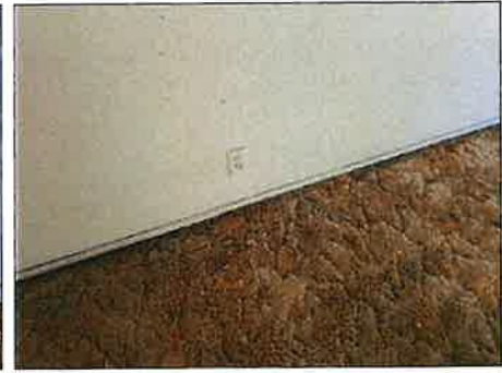
Ungrounded outlets present - typical for the age of the structure - consider upgrading electrical services
