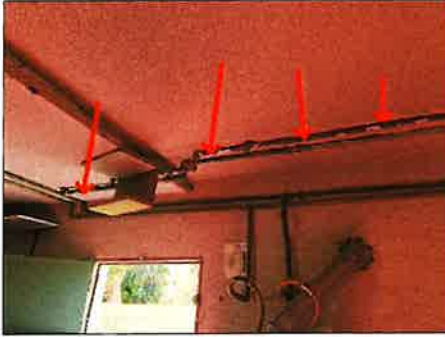
Galvanized water piping present - recommend complete evaluation of water distribution system
