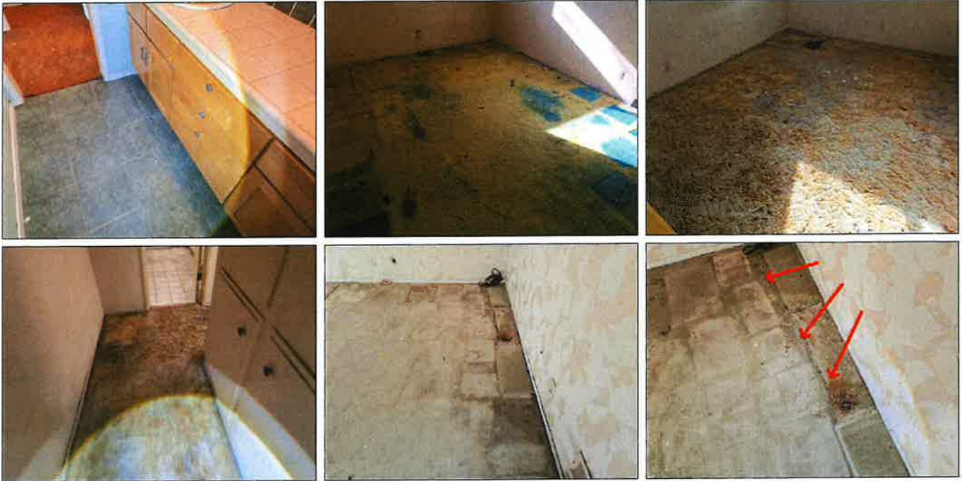
Evidence of rodents/pests - recommend pest services inspection for further evaluation
