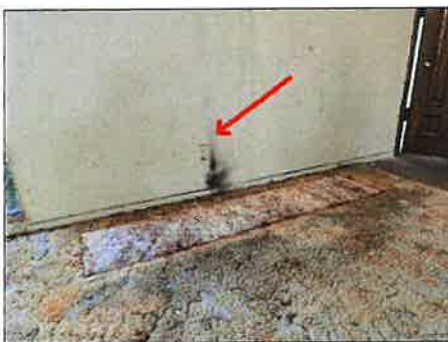
Charred/evidence of overheating at outlet(s) - needs to be serviced
