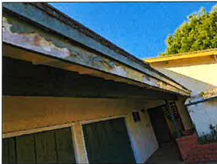
Paint deteriorated - recommend servicing
