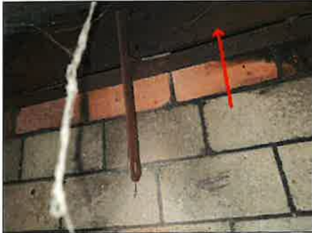
Damper door is stuck - needs to be serviced
