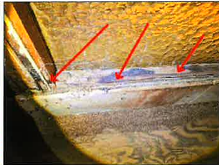
Deteriorated frames - recommend servicing
