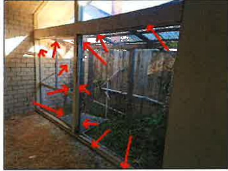
Damaged/ heavily deteriorated frames/ needs servicing and further evaluation
