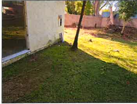
Stained areas show evidence of ponding water or poor drainage – recommend further evaluation
