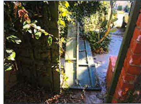
Heavily damaged - needs to be serviced
