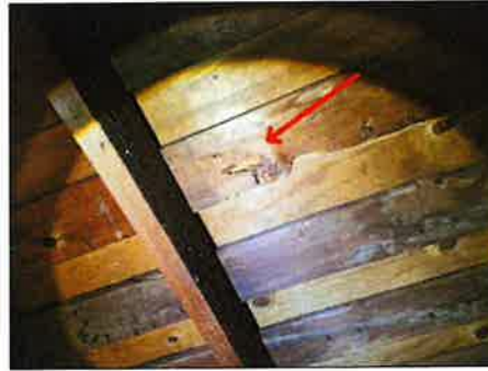
Wood deterioration observed - consult termite report for any wood areas in garage area
