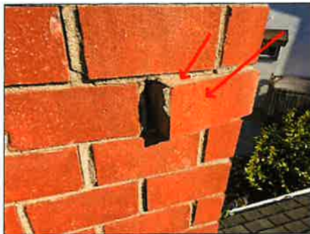
Loose bricks/mortar - needs to be evaluated by a CSIA or other certified chimney sweep
