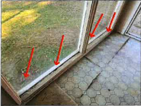
Deteriorated frame(s)- needs to be serviced
