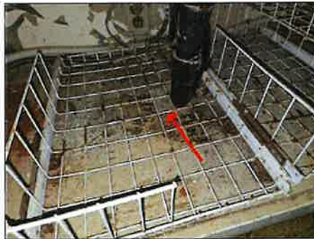
Visible leaking under sink - recommend licensed plumbing contractor for further evaluation and repair
