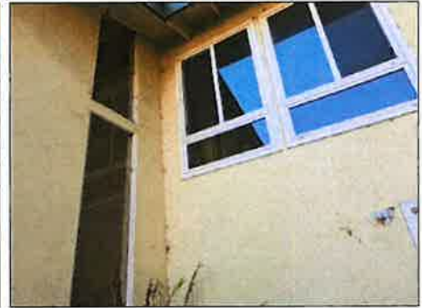
Deteriorated frames - needs to be serviced
