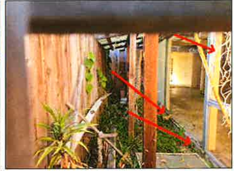
Deteriorated frames - needs to be serviced
