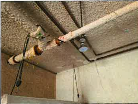
Galvanized water piping present - recommend complete evaluation of water distribution system
