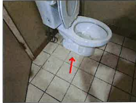
Toilet loose at floor - needs to be serviced
