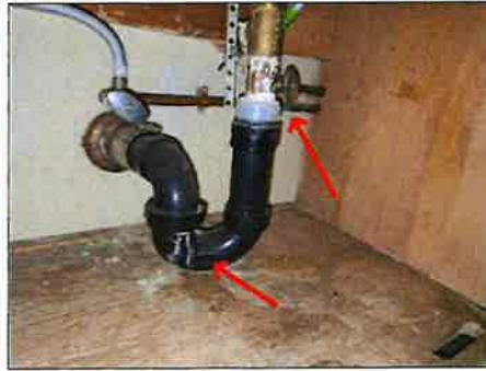
Visible leaking under sink - recommend licensed plumbing contractor for further evaluation and repair
