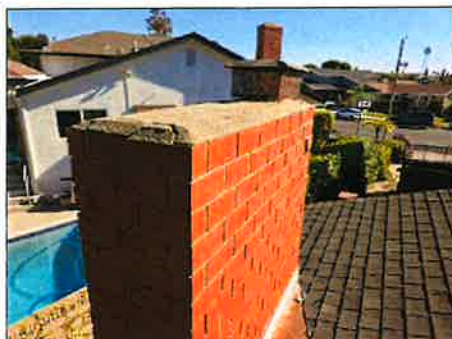
Loose bricks/mortar - needs to be evaluated by a CSIA or other certified chimney sweep
