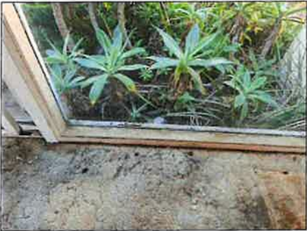
Deteriorated frame(s)- needs to be serviced
