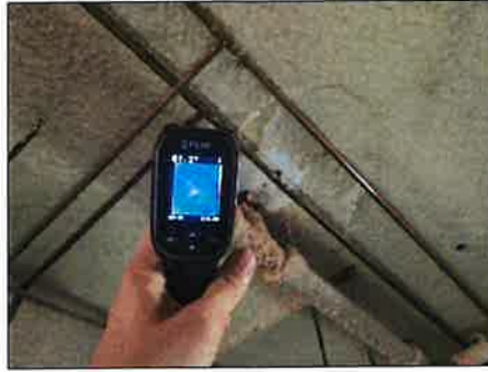
Stains present - tested dry at time of inspection - monitor for possible moisture intrusion
