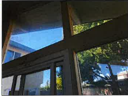
Damaged/ heavily deteriorated frames/ needs servicing and further evaluation
