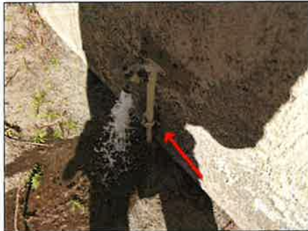
Galvanized water piping present - recommend complete water distribution system evaluation beyond the scope of this inspection due to age/type
