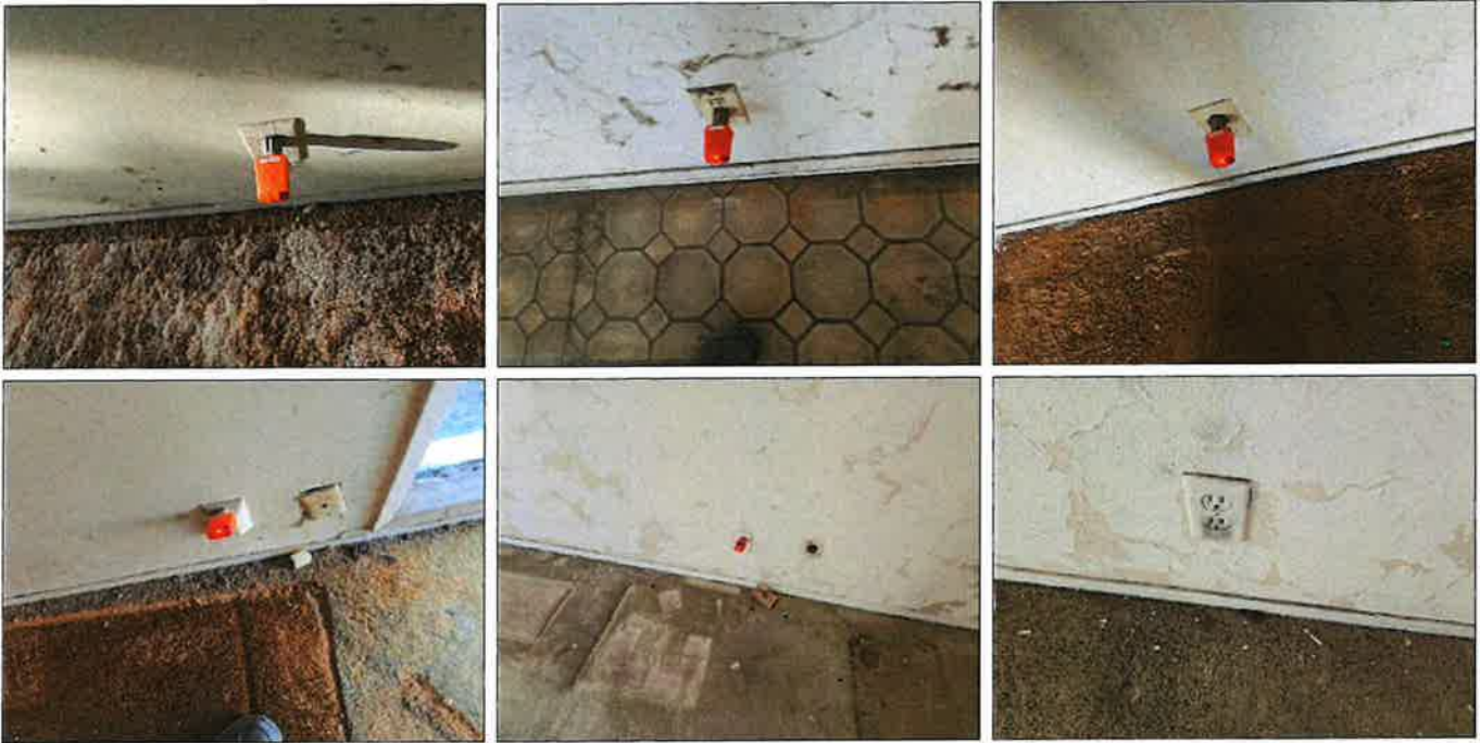
Charred/evidence of overheating at outlet(s) - needs to be serviced
