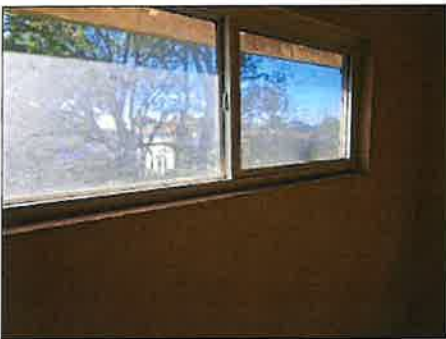
Stains/blisters at sill - tested dry for moisture at the time of the inspection - monitor the areas for moisture intrusion
