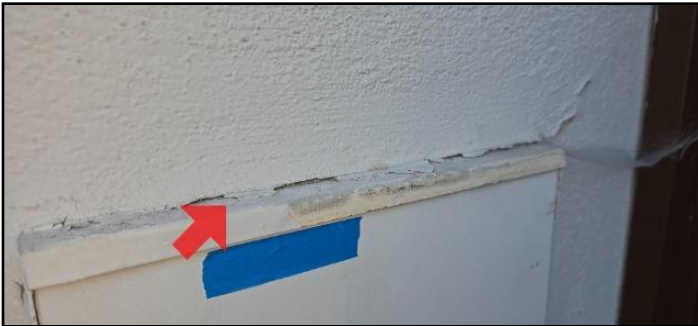
7. Minor cracks
