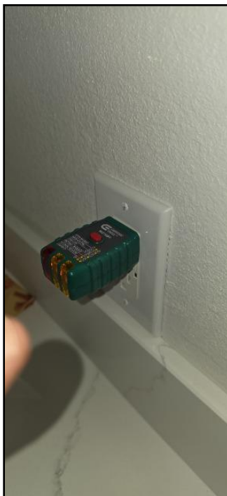
16. Arc Fault Circuit Interrupter (AFCI) test...
