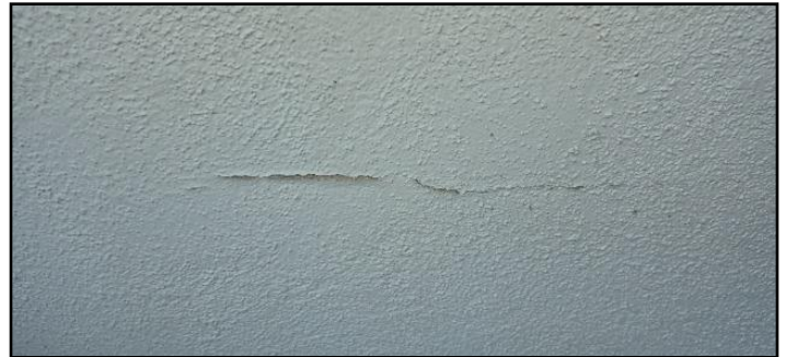
8. Minor cracks
