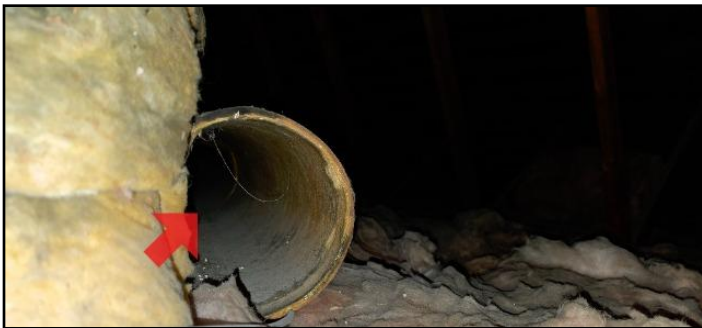
21. Disconnected ducts
