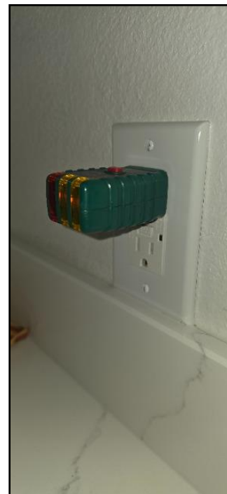
17. Arc Fault Circuit Interrupter (AFCI) test...
