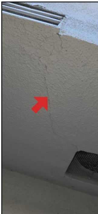
9. Minor cracks
