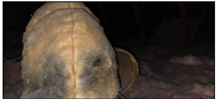
22. Disconnected ducts
